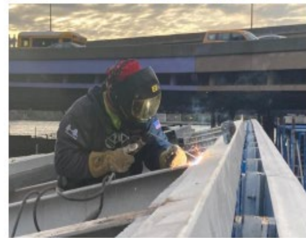
Construction of interceptor gate building – October 2025
