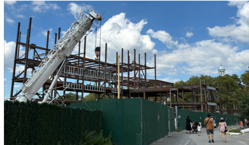
Construction Looking North
