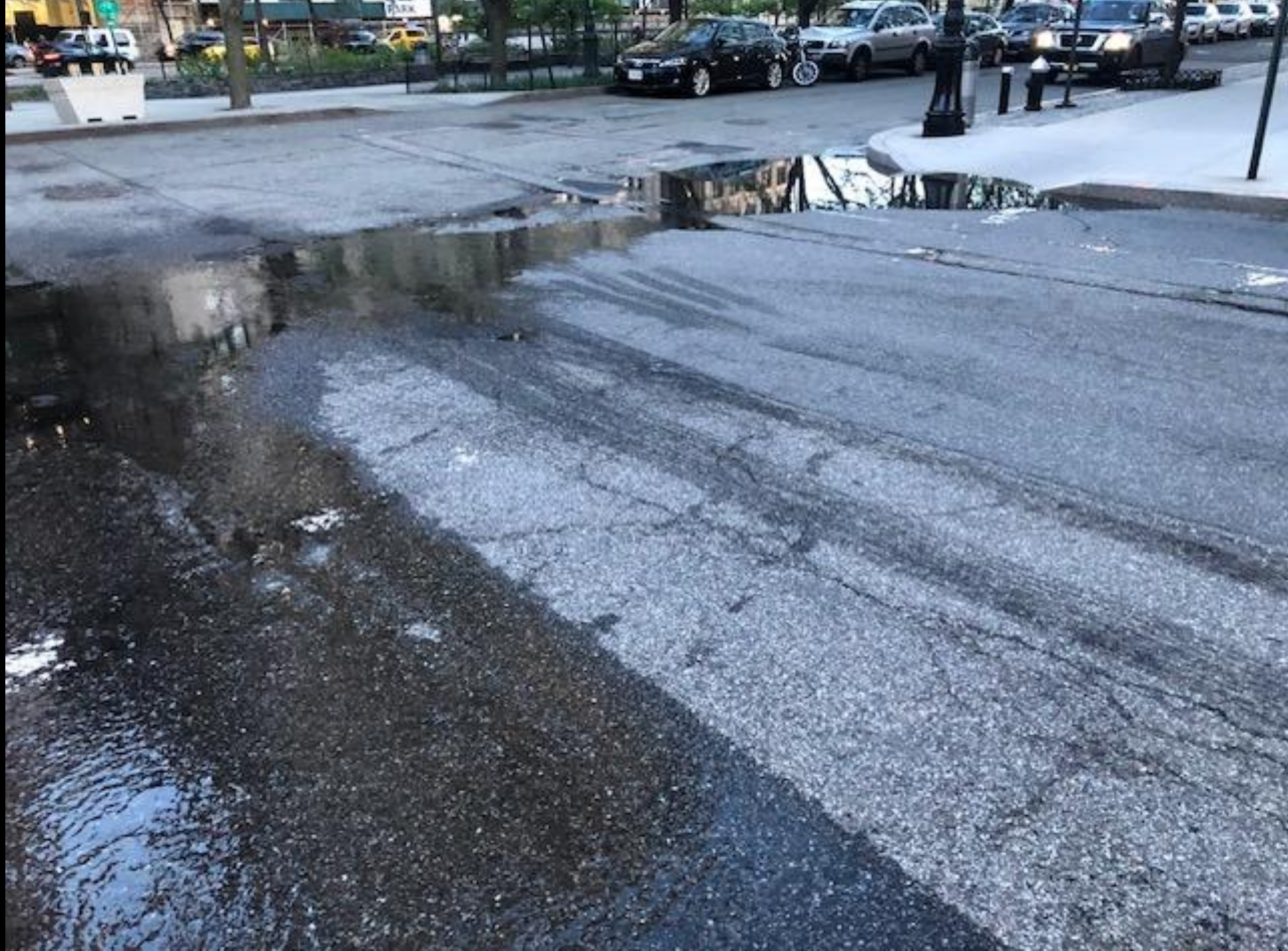
Ponding on 2nd Pl at Little West St
