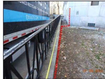
PHOTO #8 - FENCE POSTS SHALL BE INSTALLED THE PLANTED AREA ALONG SIDE THE EXISTING FENCE CURB. PLEASE CONFIRM THAT THE FENCE IS NOT INSTALLED ALONG THE SIDE OF THE BUILDING BUT STOPS AT THE BUILDING AS SHOWN.
