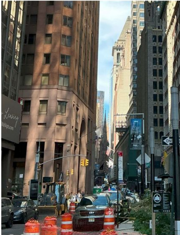
Location of proposed 95 Wall Street 5G tower site from the east looking west on 09-24-24.
