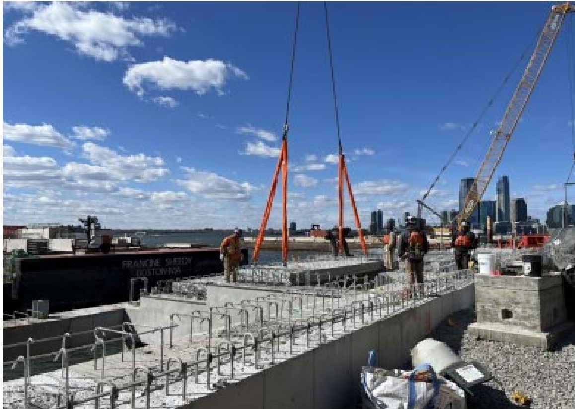
February 2025 – Precast Plank Installation
