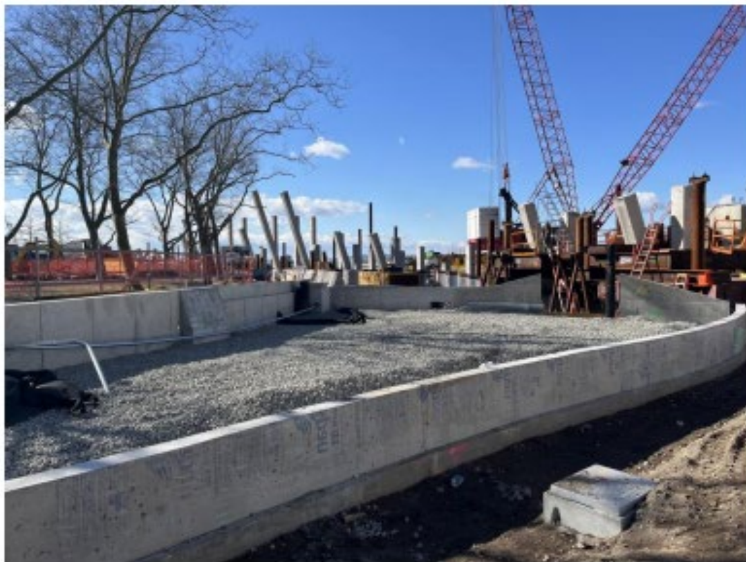
February 2025 – Placement of Ultra Lightweight Foam Glass Aggregate Fill
