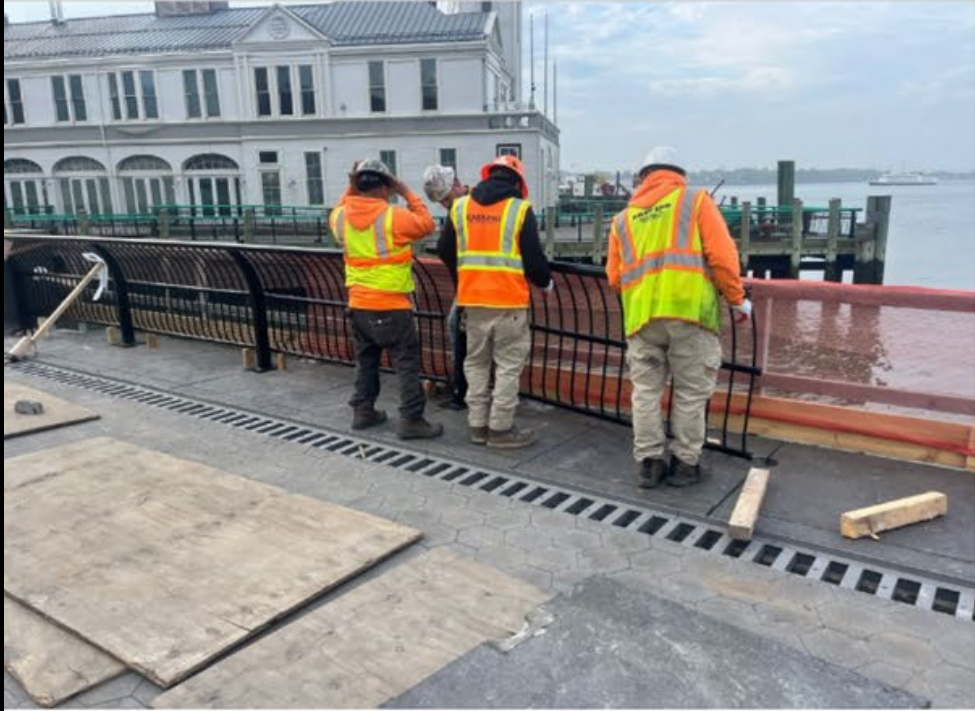
Esplanade railing installation and Pier A inlet progress
