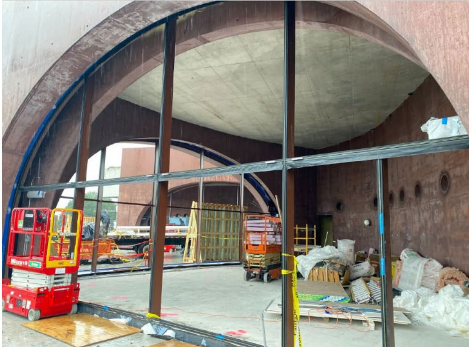
Stone installation along Battery Place, and curtain wall installation in the pavilion
