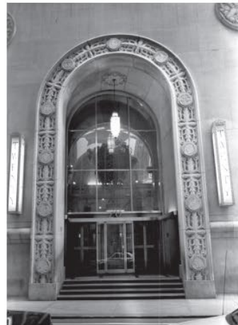
replaced lantern fixture replaced arch glazing and entrance storefront new illuminated signage
