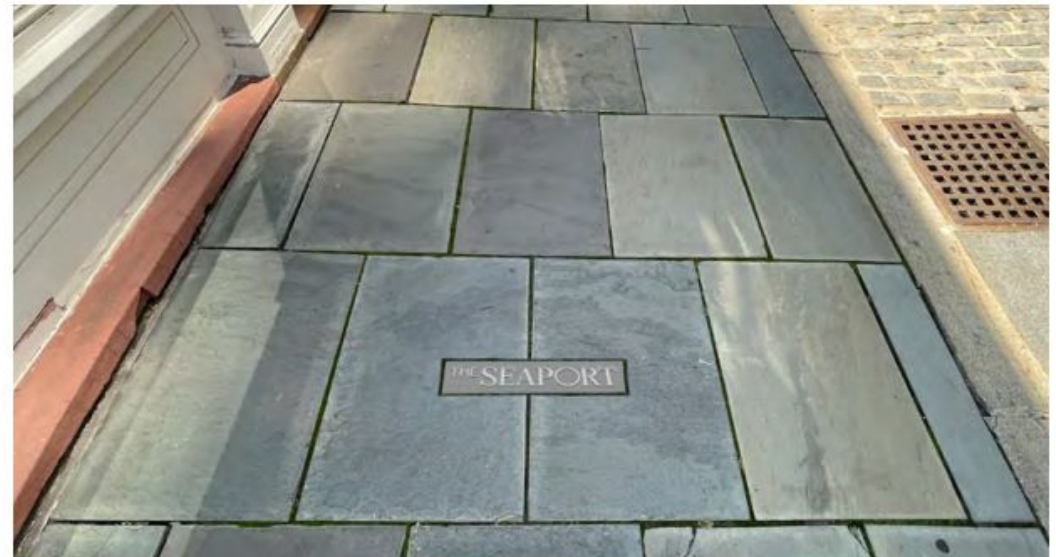
Sign A3, Quantity 12, Reversed Etched Zinc to simulate Stainless Steel
