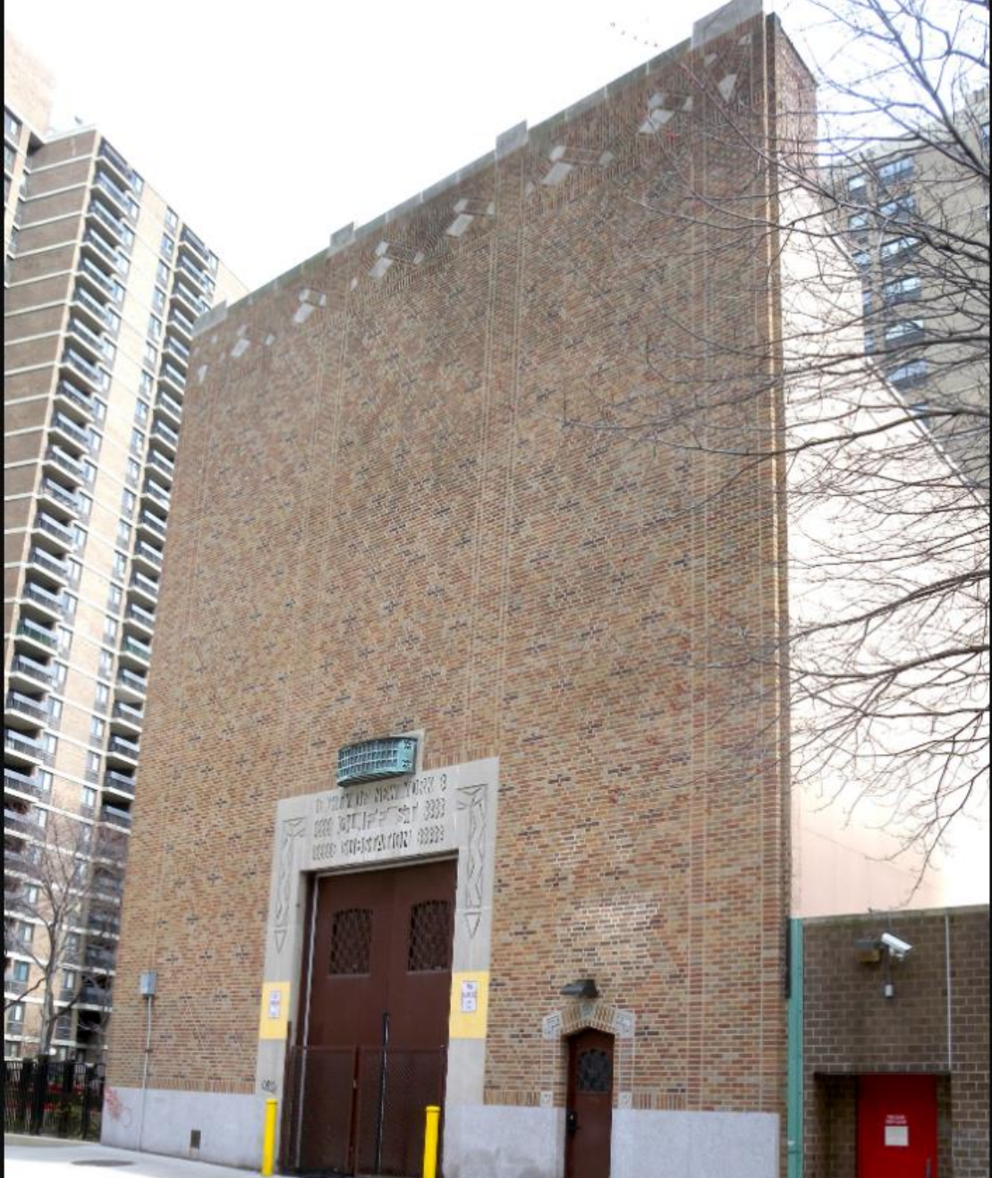
CLIFF STREET STATION @ SOUTHBRIDGE
