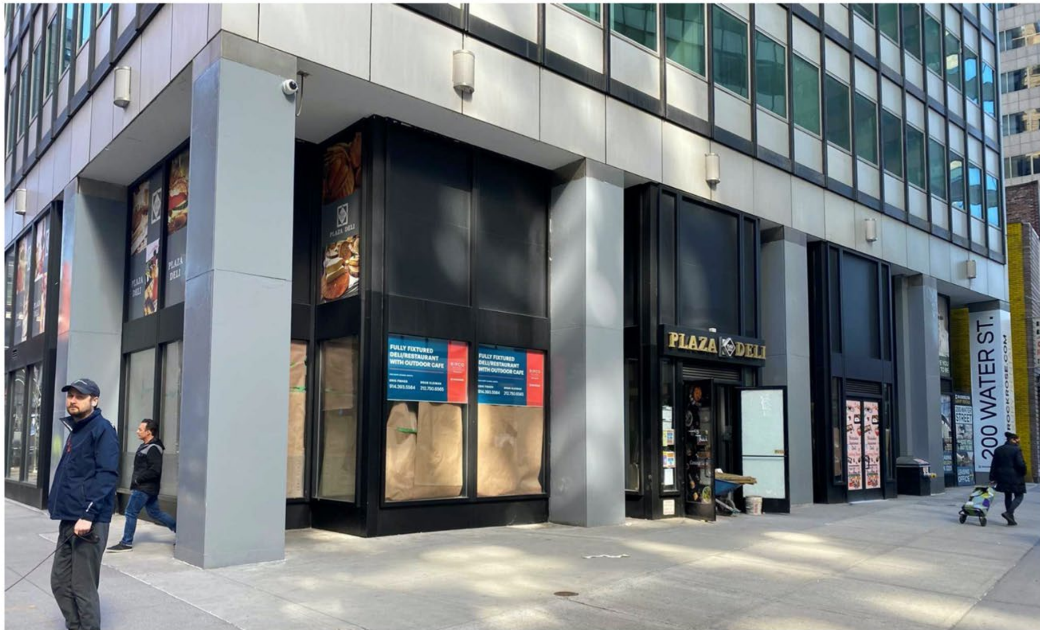
JOHN STREET PLAZA - EXISTING CONDITIONS
