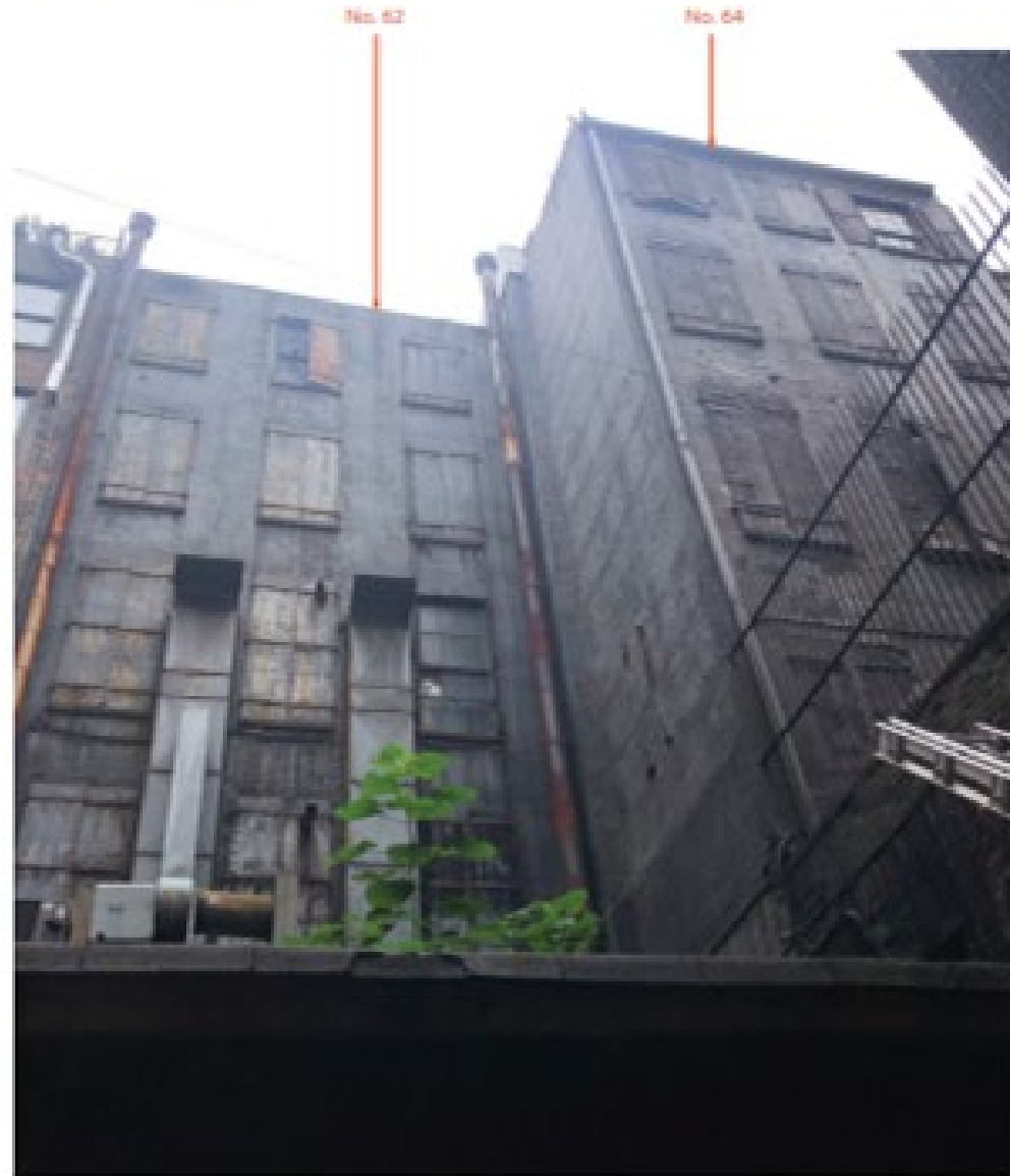
Rear elevation from courtyard (facing south)
