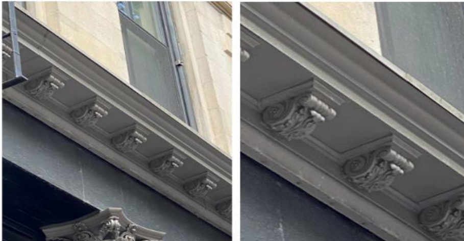
3 ENLARGED PHOTOS OF 38 WALKER NEW FIBERGLASS CORNICE
