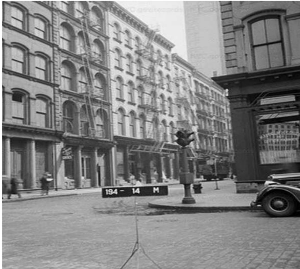
1940'S TAX PHOTO - FRONT FACADE
