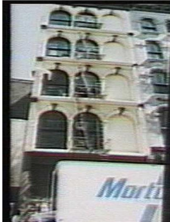
1980'S TAX PHOTO - FRONT FACADE
