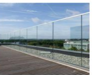
8_GLASS RAILING COLOR FINISH: LOW IRON GLASS wNON-REFLECTIVE COATING SAMPLES WITH BE PROVIDED TO LPC FOR APPROVAL
