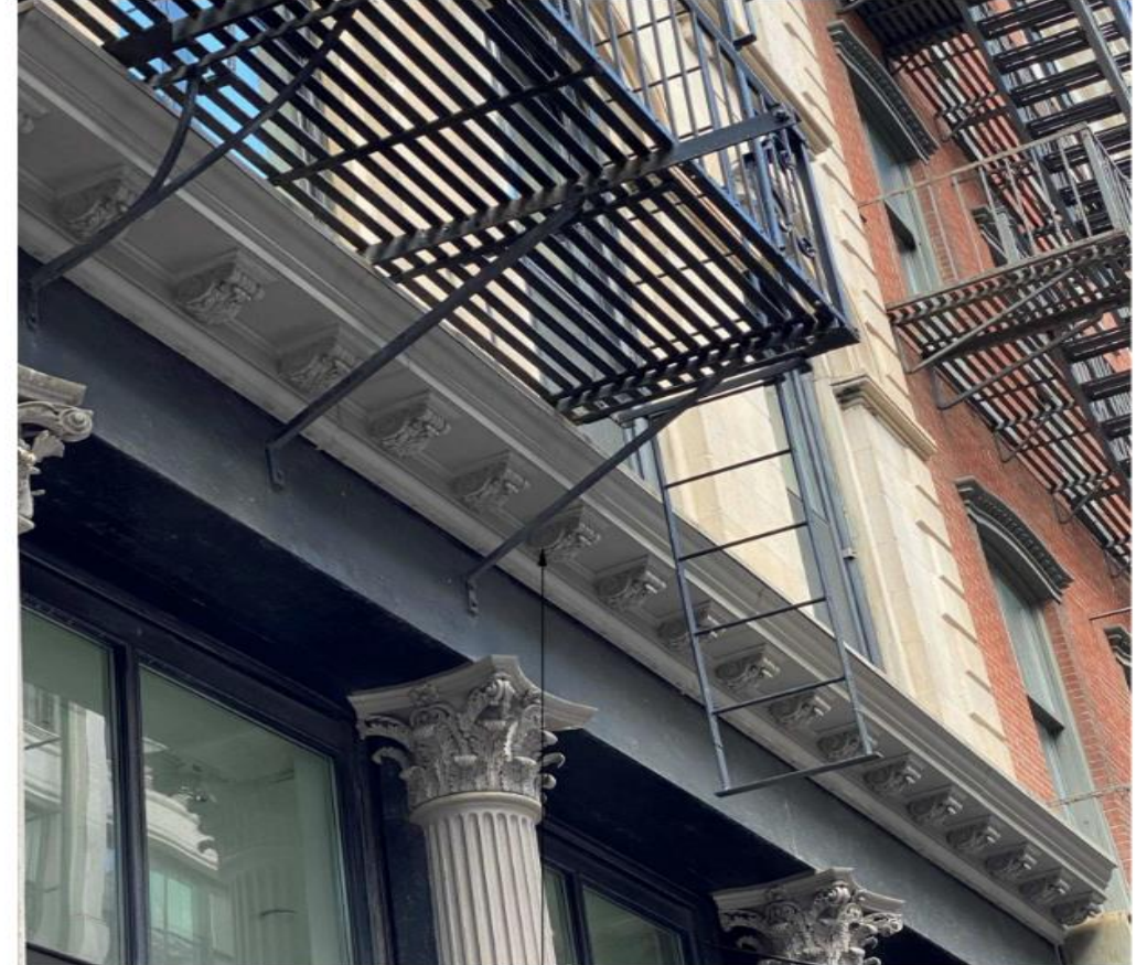
2_38 WALKER - NEW FIBERGLASS CORNICE
