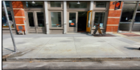
2 EXISTING SIDEWALK PHOTO AT ADJACENT SIDEWALK
