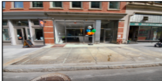
4 EXISTING SIDEWALK PHOTO
