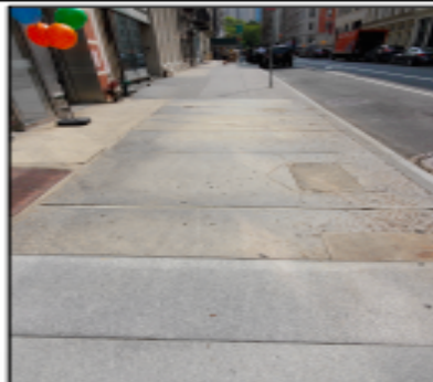
7 EXISTING SIDEWALK PHOTO
