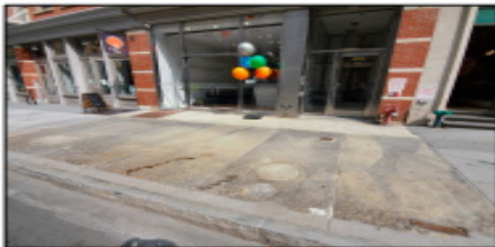
6 EXISTING SIDEWALK PHOTO
