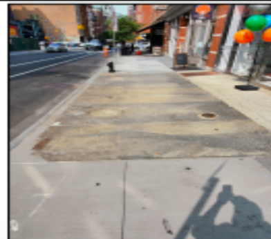
8 EXISTING SIDEWALK PHOTO
