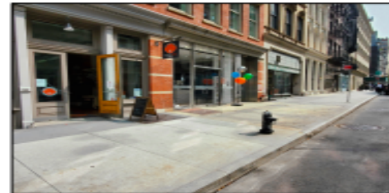
5 EXISTING SIDEWALK PHOTO
