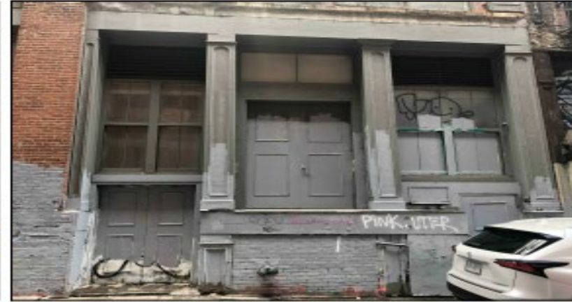
03 PHOTO AT NORTHERN—MOST WINDOW BAYS
