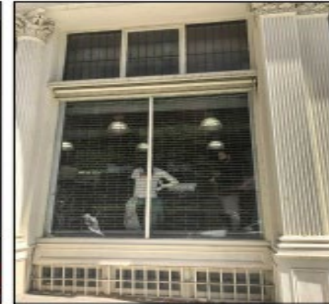
06 CELLAR CLERESTORY WINDOWS @ 380 BROADWAY
