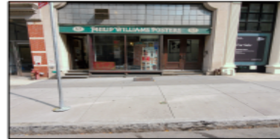
3 EXISTING SIDEWALK PHOTO AT ADJACENT SIDEWALK
