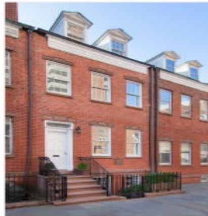
EXISTING FACADE ● 31 HARRISON ST NTS ⑤
