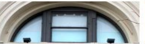
EXISTING WINDOW FRAME FINISH TO REMAIN
