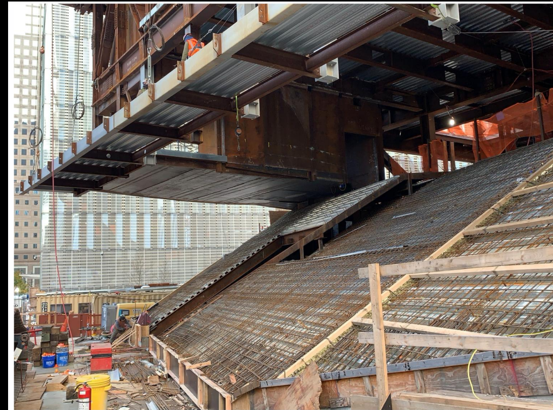
December 2020: Grand Staircase begins to take shape under the cantilever.
