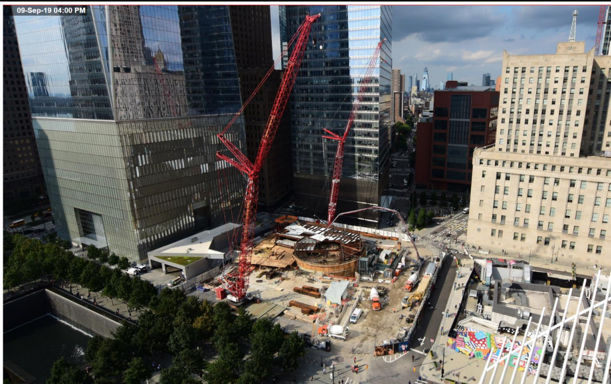
September 9, 2019: Both the North and South TPC cranes are erected and become operational as the Port Authority WBVA* structure continues below. *West Bathtub Vehicle Access
