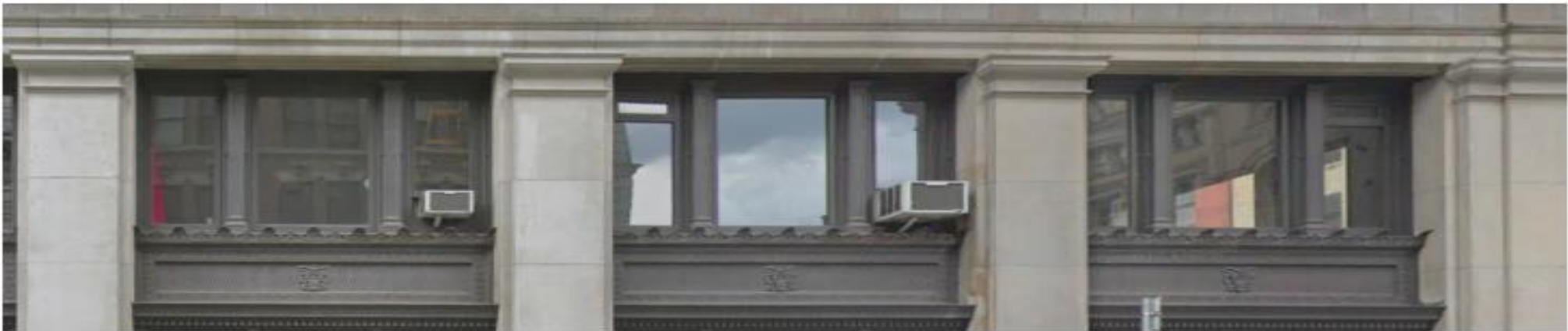
② CLOSE-UP VIEW OF EXISTING APT 2E NORTH WINDOWS
