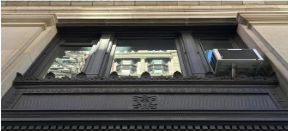
① CLOSE-UP VIEW OF EXISTING APT 2E WEST WINDOWS
