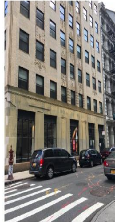
① EXISTING CONDITION PHOTOS FRANKLIN STREET FACADE
