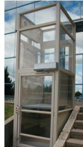
EXAMPLE OF POWDER COATED STAINLESS STEEL FRAMED LIFT WITH CLEAR GLASS PANELS
