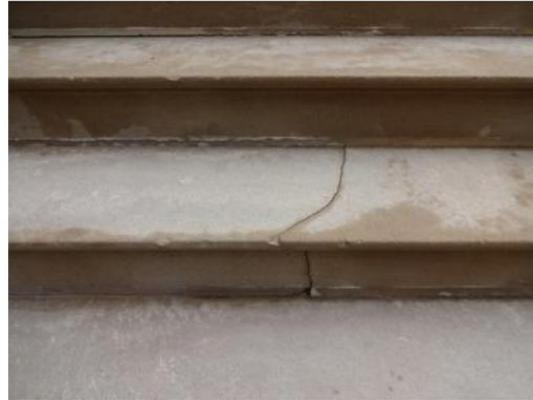
CRACKS, DETERIORATED MORTAR JOINTS, UNEVEN COATING
