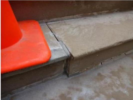
DISPLACED AND SHIFTED TREADS WITH DETERIORATED MORTAR
