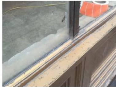
EXISTING 13 PARK ROW SILL
