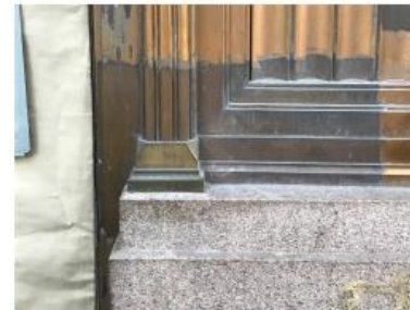
EXISTING TYPICAL PILASTER
