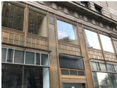
EXISTING 13 PARK ROW TRANSOM
