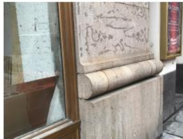
EXISTING STONE COLUMN AT 13 PARK ROW
