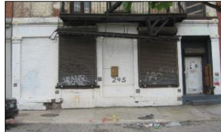
1 EXISTING STOREFRONT PHOTO (BEFORE)
