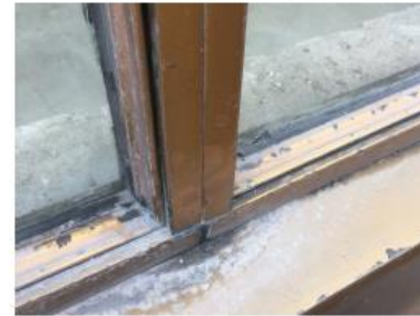
EXISTING 13 PARK ROW WINDOW MULLION
