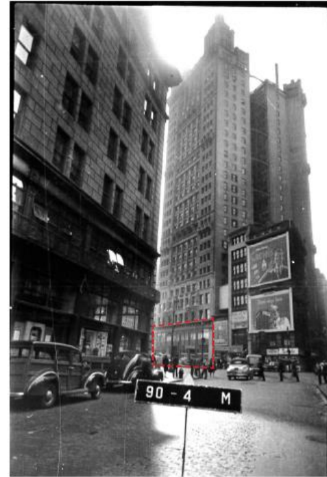
1940'S TAX PHOTO AFTER THE 1930'S STOREFRONT ALTERATION
