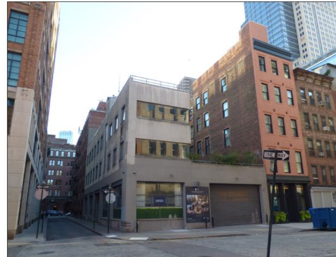
11 Hubert Street, Existing
