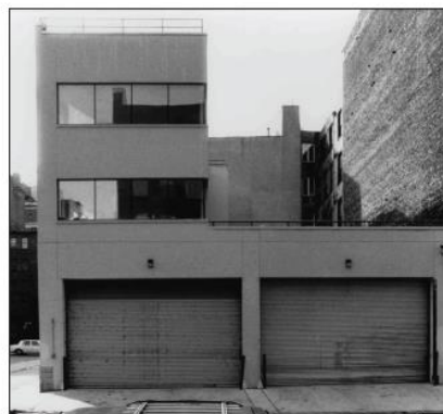
1991: 11 Hubert - Garage & Offices (Unknown, 1990) (LPC Designation Photos)
