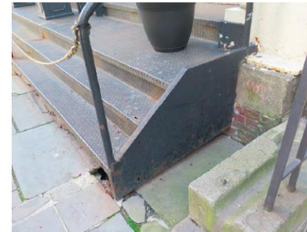
EXISTING STAIR DETAIL PHOTOGRAPH AT SIDEWALK
