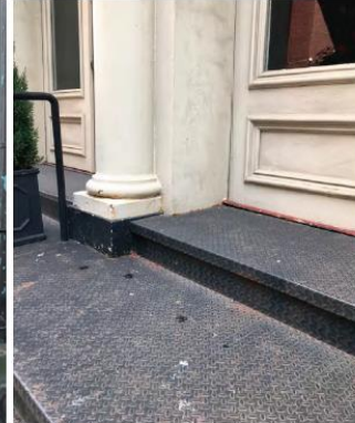
Threshold of Entry Doors
