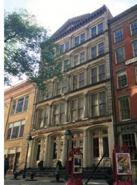
Exterior Facade at Water Street
