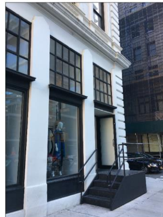
EXIST. CHURCH STREET STOREFRONT: TENANT B ENTRANCE
