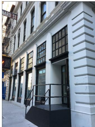
EXIST. CHURCH STREET STOREFRONT: TENANT B ENTRANCE
