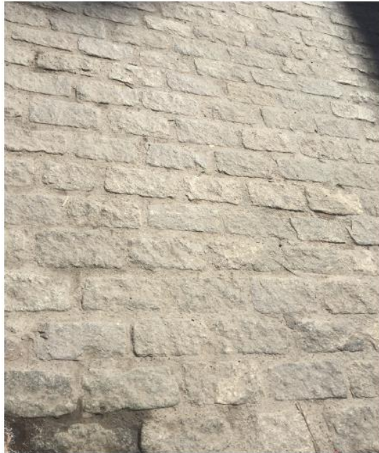
Grout flush with surface, cobbles aligned, ADA-accessible
