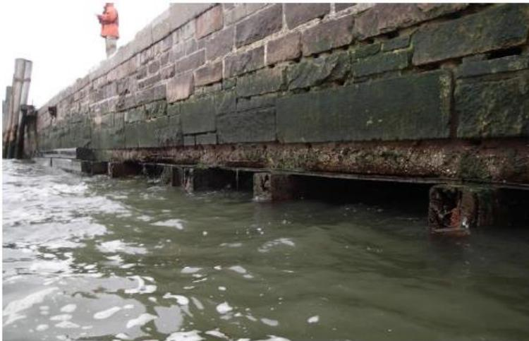
*View from water showing deteriorated wall conditions*
