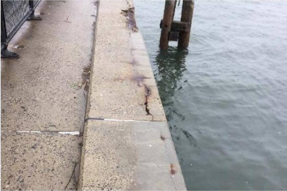
*Cracking, spalling concrete, exposed rebar*
