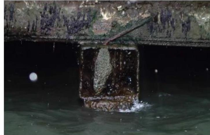
*Deteriorating timber pile caps*
