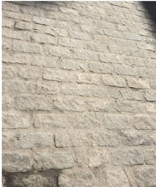
Grout flush with surface, cobbles aligned, ADA-accessible
