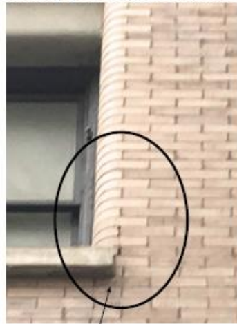
EXISTING CONDITION -Location C
