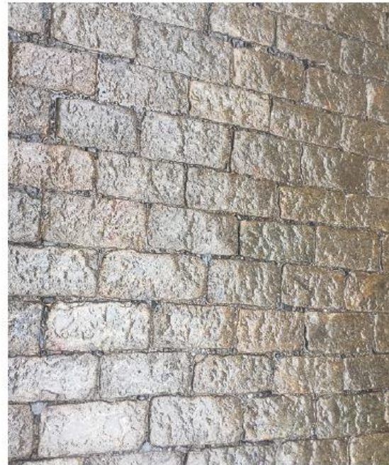
Cobbles aligned, small joints, grout (mostly) flush with surface
