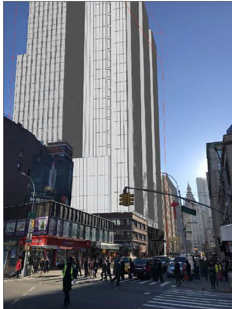
View south from Centre Street and Canal Street
