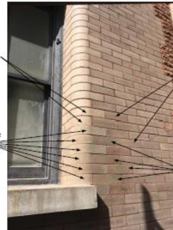
MOCK-UP SAMPLE REPAIR -Location C
