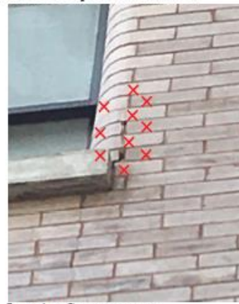
Location C - 3rd floor window
