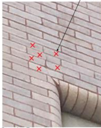
Location B - 2nd floor window
