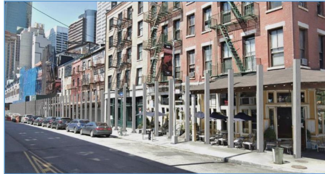
12-ft high posts to hold stop logs
