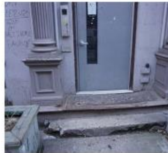
EXISTING 105 READE ENTRANCE CONDITION
