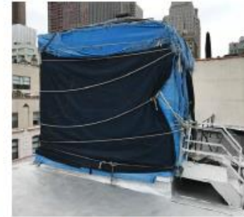
EXISTING ROOFTOP BULKHEAD CONDITION
