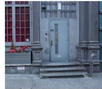
EXISTING 107 READE ENTRANCE CONDITION
