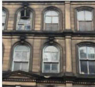
EXISTING FACADE & WINDOW CONDITION
