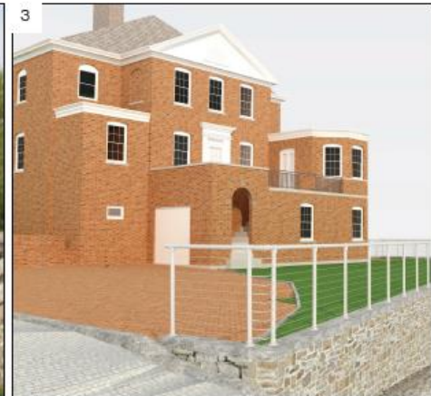
Rendering of proposed pipe hand rail and coping stone.
