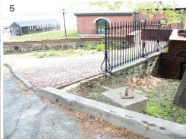
5 (2018) View of lower retaining wall at Barry Road.
