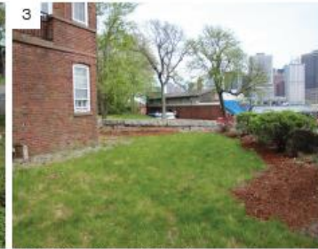
3 (2018) View of inboard side of upper wall
