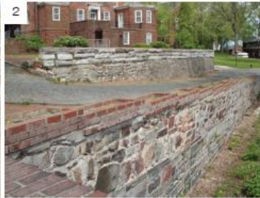
2 (2018) View of lower and upper wall
