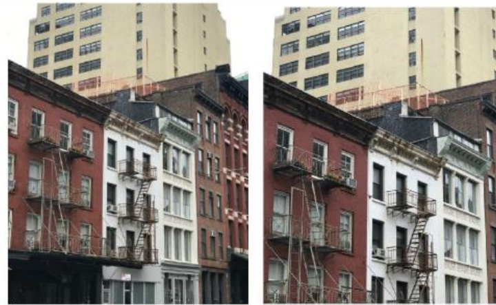
MOCK-UP CLOSEUP VIEW FROM THE CORNER OF HARRISON & GREENWICH ST
