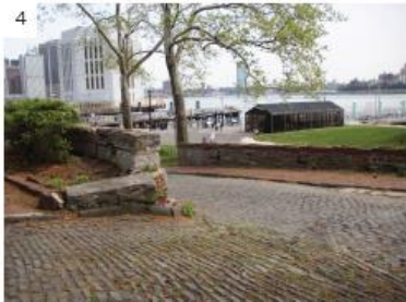
4 (2018) View of inboard upper and lower wall from cobblestone driveway.
