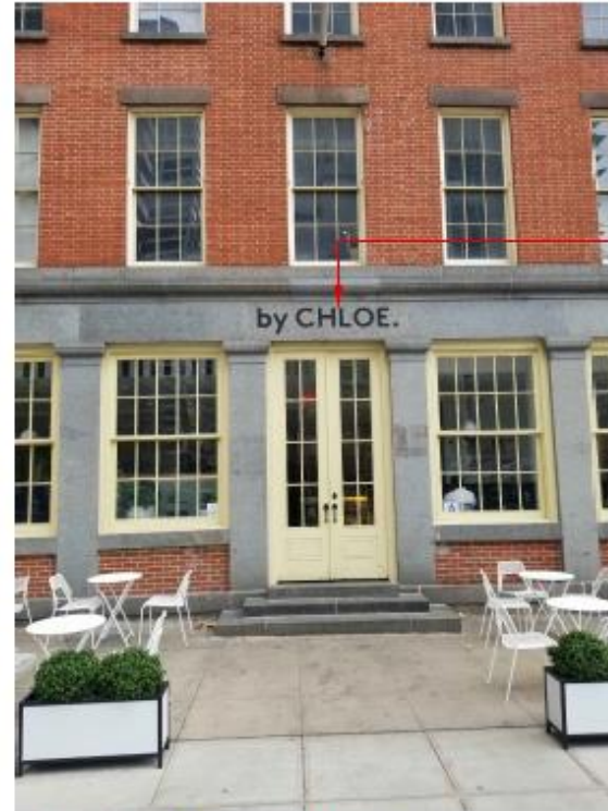
2 Existing Condition Photographs - John Street
