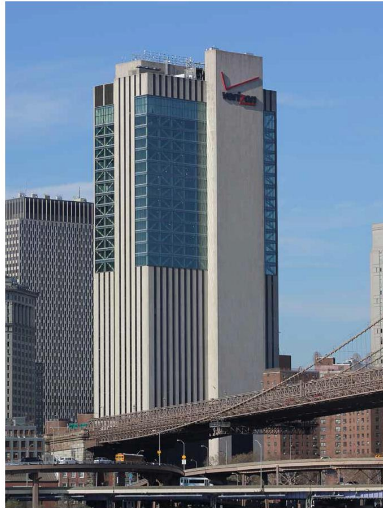
2 EXISTING VERIZON SIGN
