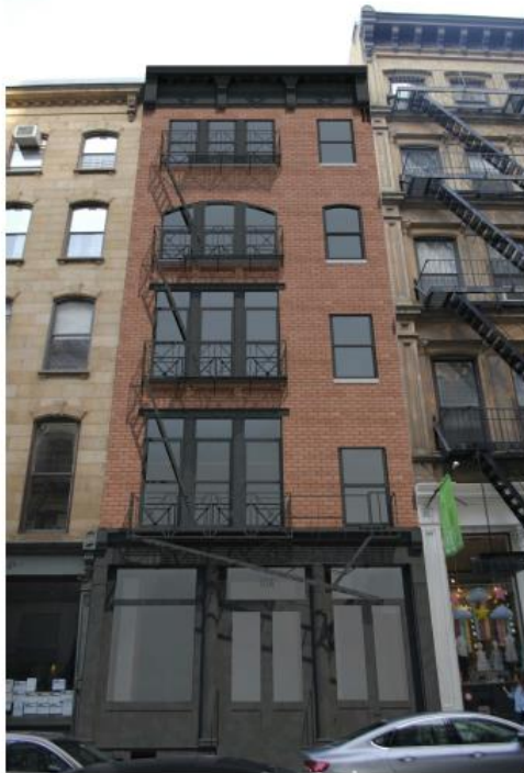
EXISTING FIRE ESCAPE
