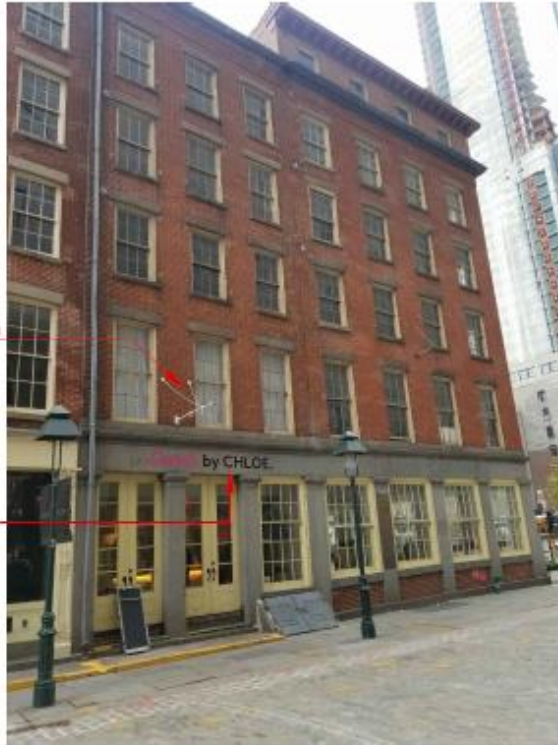
1 Existing Condition Photographs - Front Street
