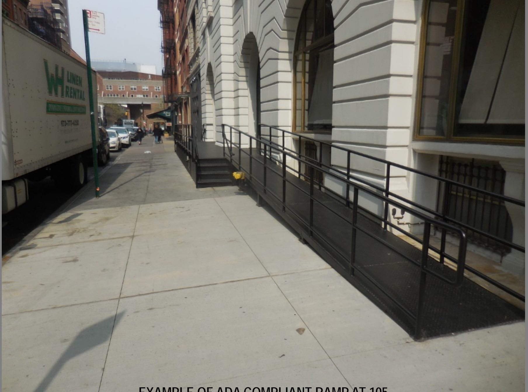
EXAMPLE OF ADA COMPLIANT RAMP AT 105 HUDSON STREET
