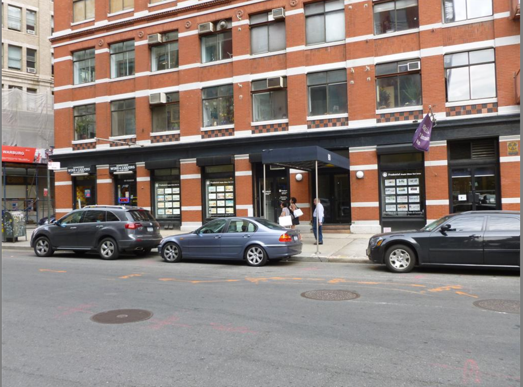
WEST ELEVATION ALONG HUDSON STREET (VIEW FACING NORTH-EAST)
