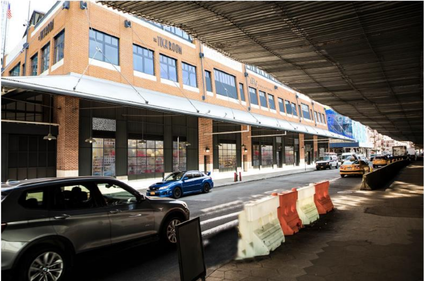
FULTON MARKET BUILDING // South Street Elevation
