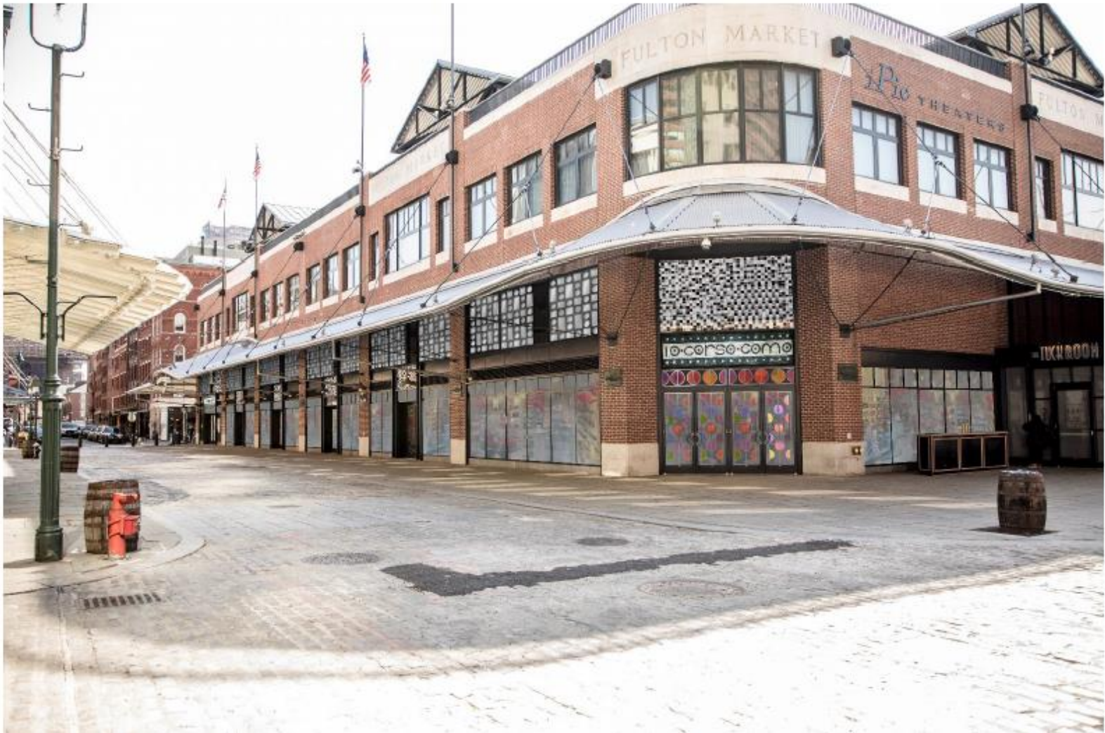
FULTON MARKET BUILDING // Front Street Elevation
