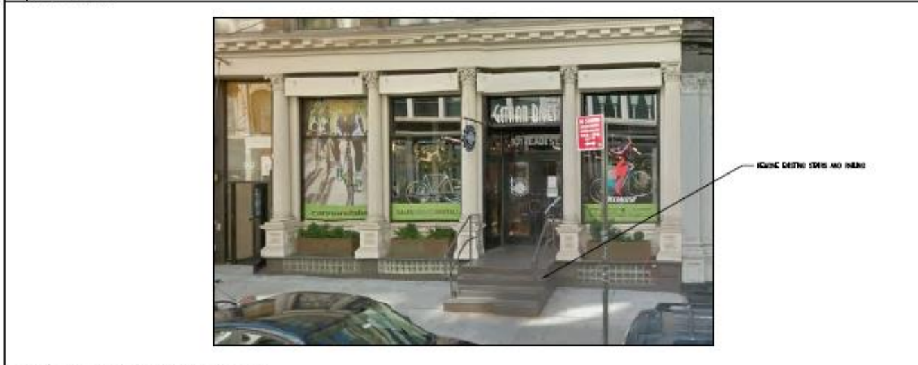
1 EXISTING EXTERIOR STAIRS - STREET VIEW - 110 READE STREET SCALE: NOT TO SCALE
