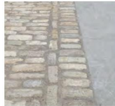
EXAMPLE OF GRANITE PAVERS SET AMONG REUSED GRANITE COBBLESTONE BLOCK
