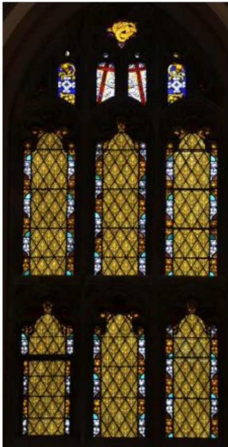
Existing window - lancets 1967, traceries 1845
