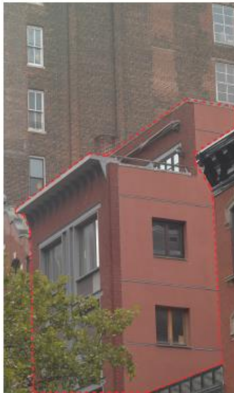
EXISTING VIEW #1 FROM DUANE STREET (ENLARGED)
