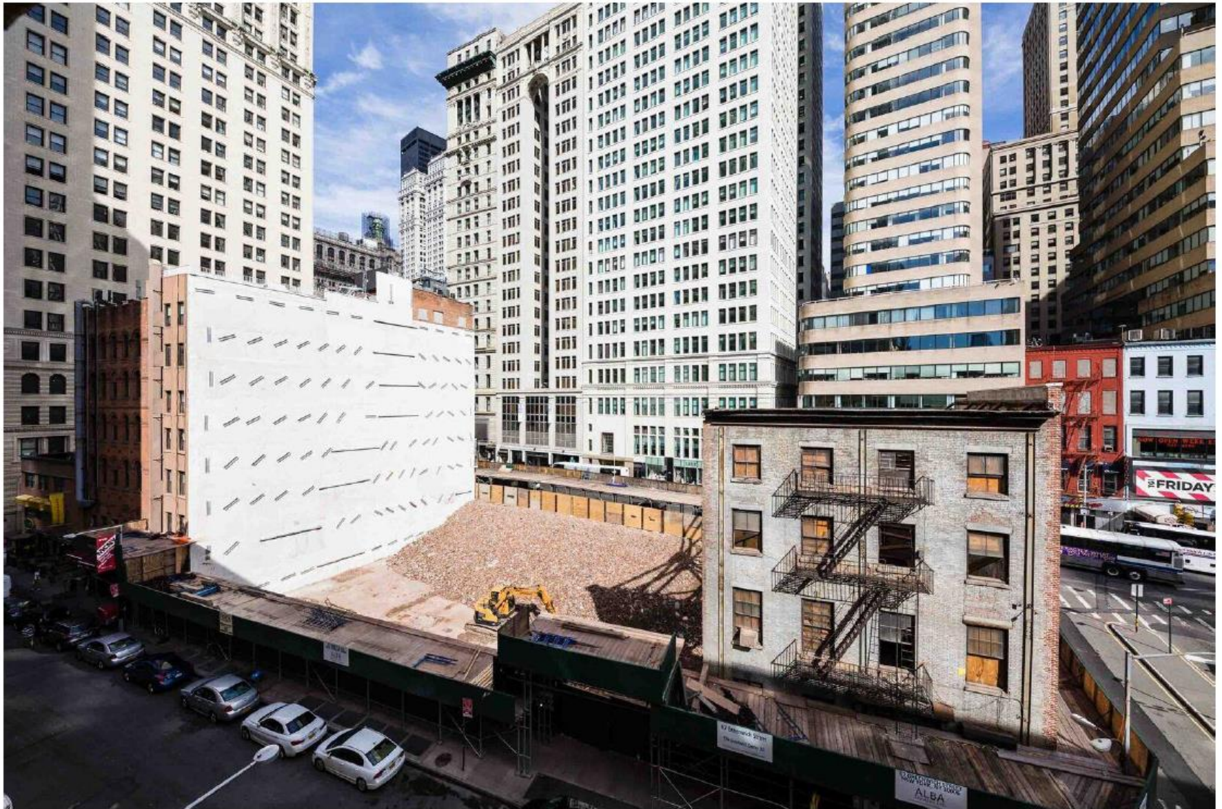
View from the Battery Parking Garage, looking east towards Broadway (Landmark façade in foreground)
