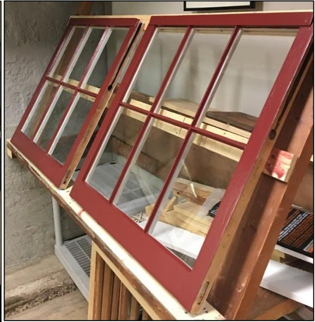
**Glazing Putty:** When you see signs of glazing putty failure, it is important to remove deteriorated sections and install new glazing putty and paint accordingly.
