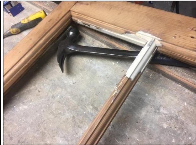
**Dutchman's:** Where signs of rot occur, it is important to remove the deteriorated section and install a dutchman. This can be done with wood or alternative materials such as epoxy.
