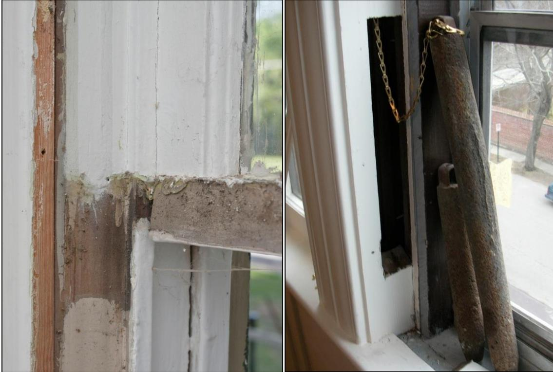
**Operation:** Cutting the paint seal, while replacing the sash cords/chains will increase the functionality of your windows. Before and after example below.
