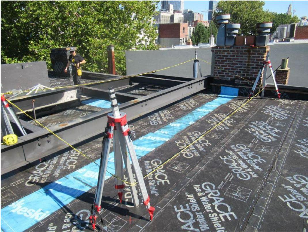
**Figure 3:** This is an example of a flat roof installation mock-up, using tripods and rigid construction tape lines to represent the size, placement, and height of the proposed installation. With this in place, applicants should then take a series of photos from surrounding public thoroughfares to document visibility.
