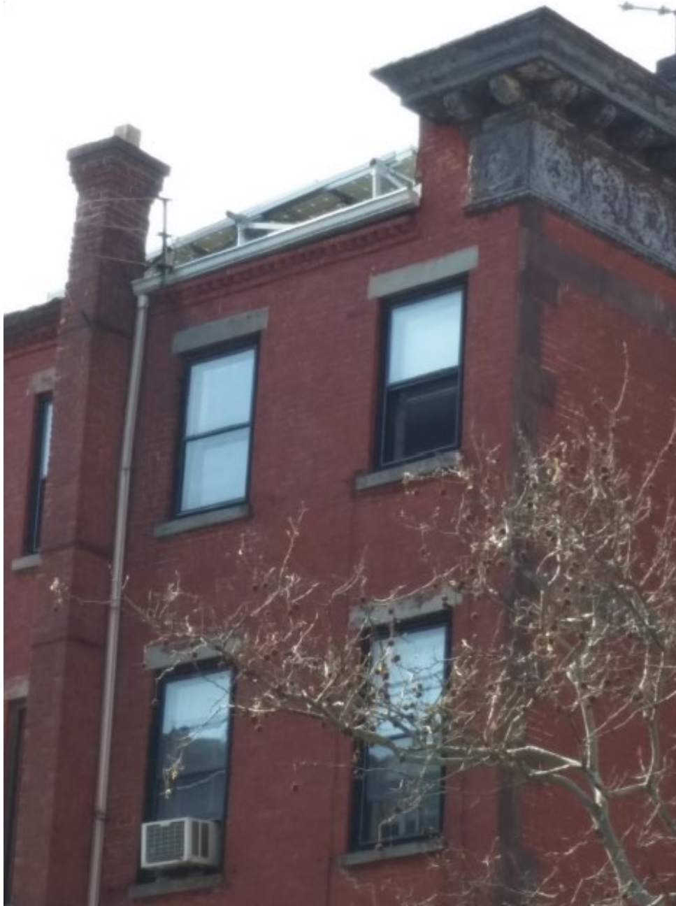
Figure 2: Solar panel installation "A" zoomed in.
