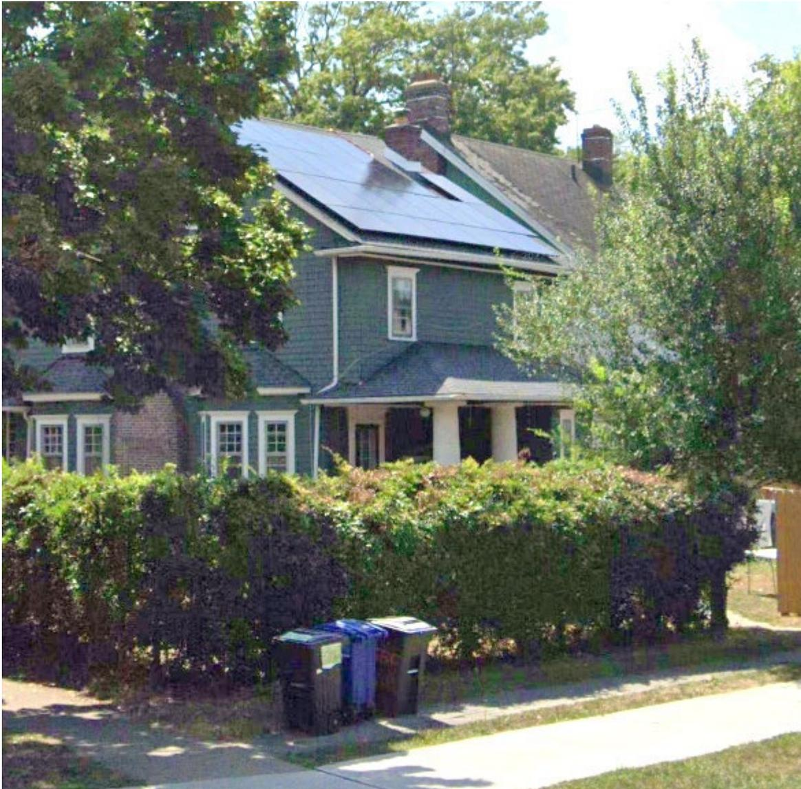
**Figure 7:** This shows an example of panels visible over a secondary façade. The panels are in a simple configuration, are mounted close to the roof surface, and follow the slope of the roof.
