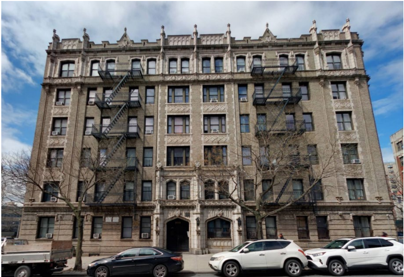
935 St. Nicholas Avenue, Cyclomedia
