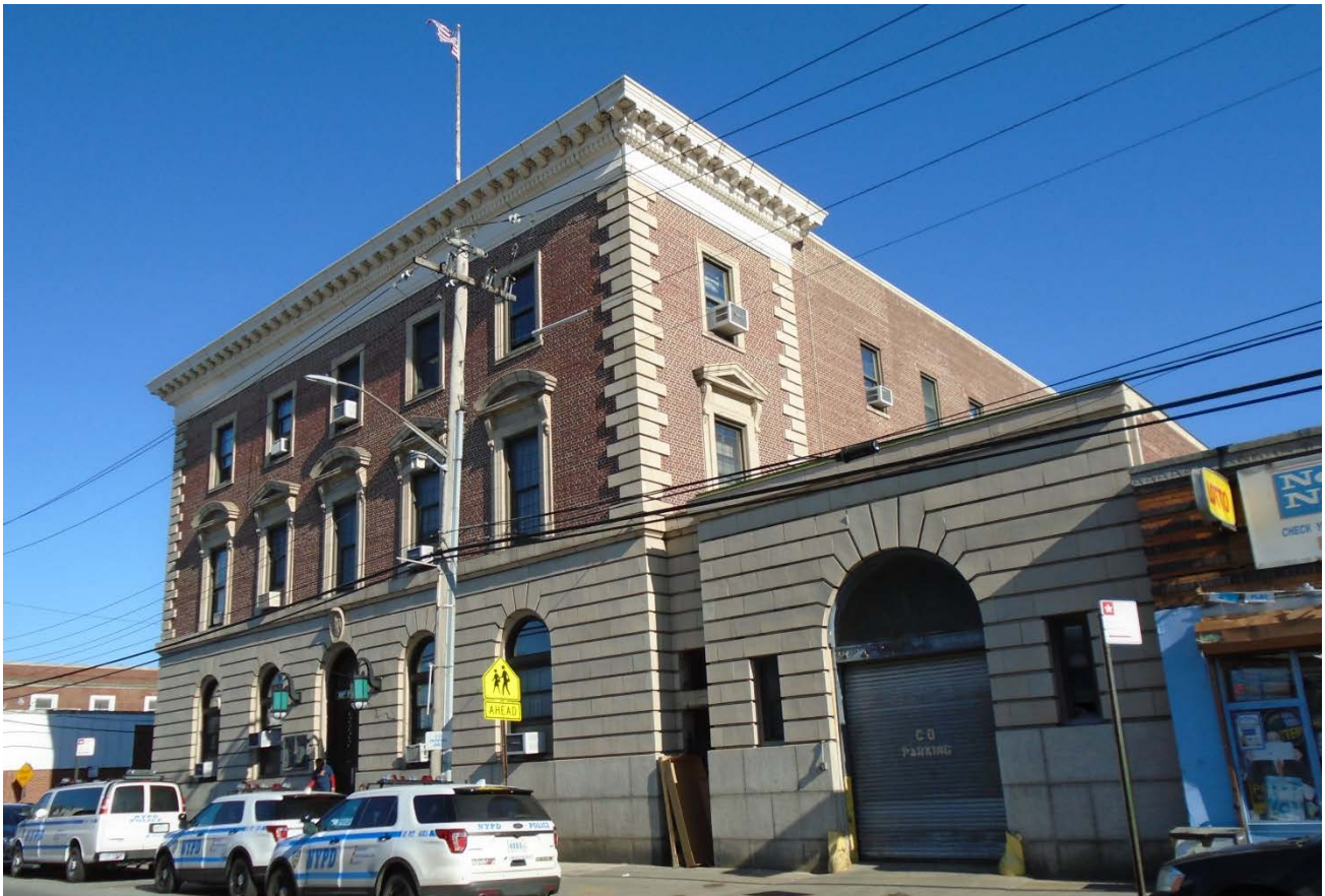
53rd (now 101st) Precinct Police Station and Garage, Mott Avenue Facade, LPC, 2018
