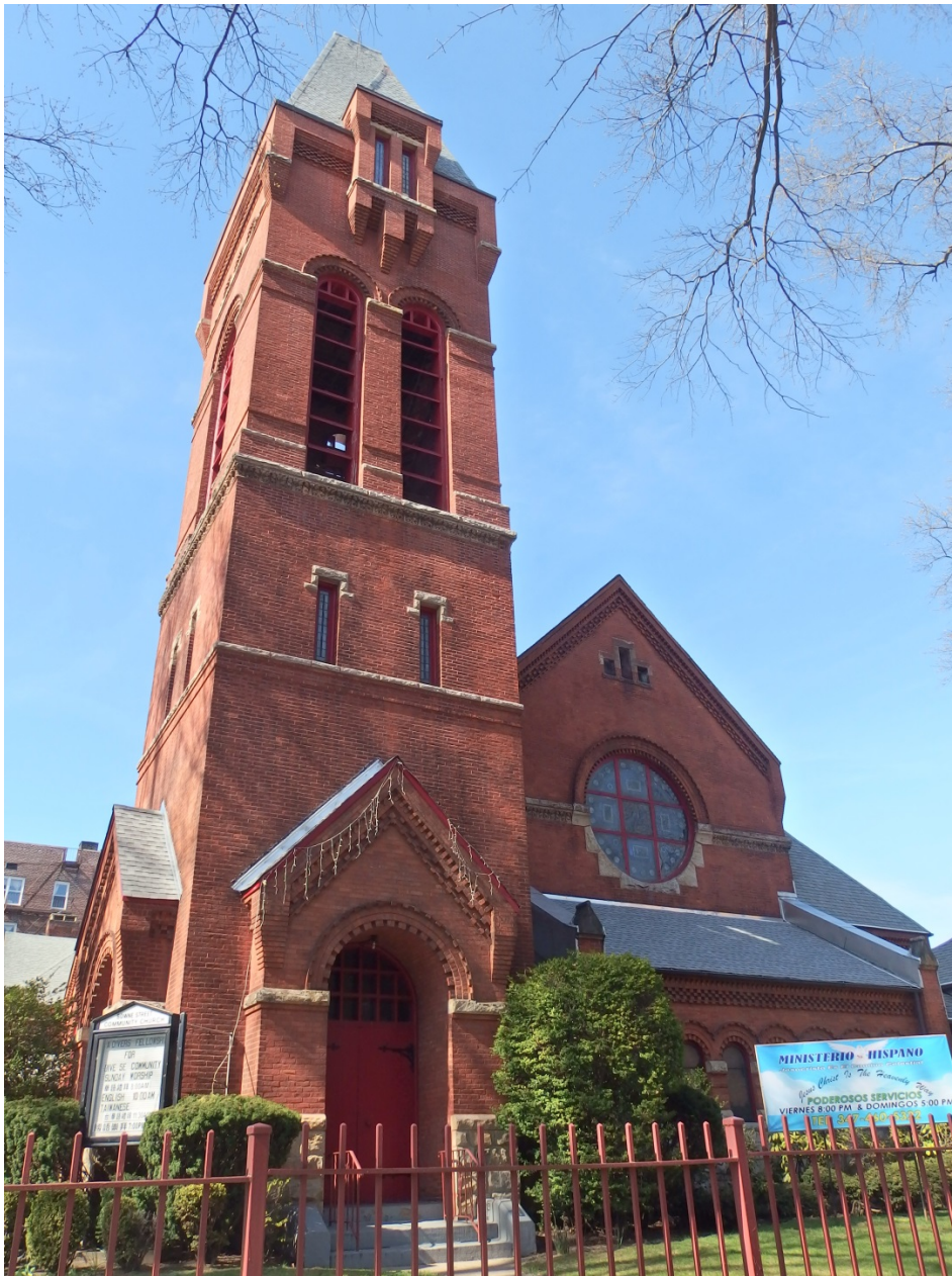
Front (south) Facade along Roosevelt Avenue
