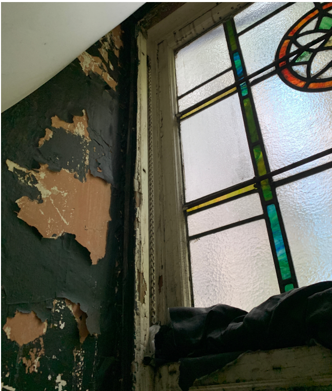
Detail of PHN (Register 1) showing watermarks on the interior of the sash and chipping paint.
