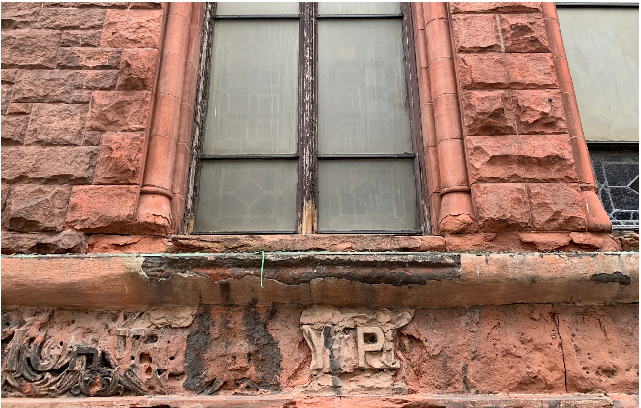
Stone spalling and delamination on the exterior of the West facade. The window sills have eroded.
