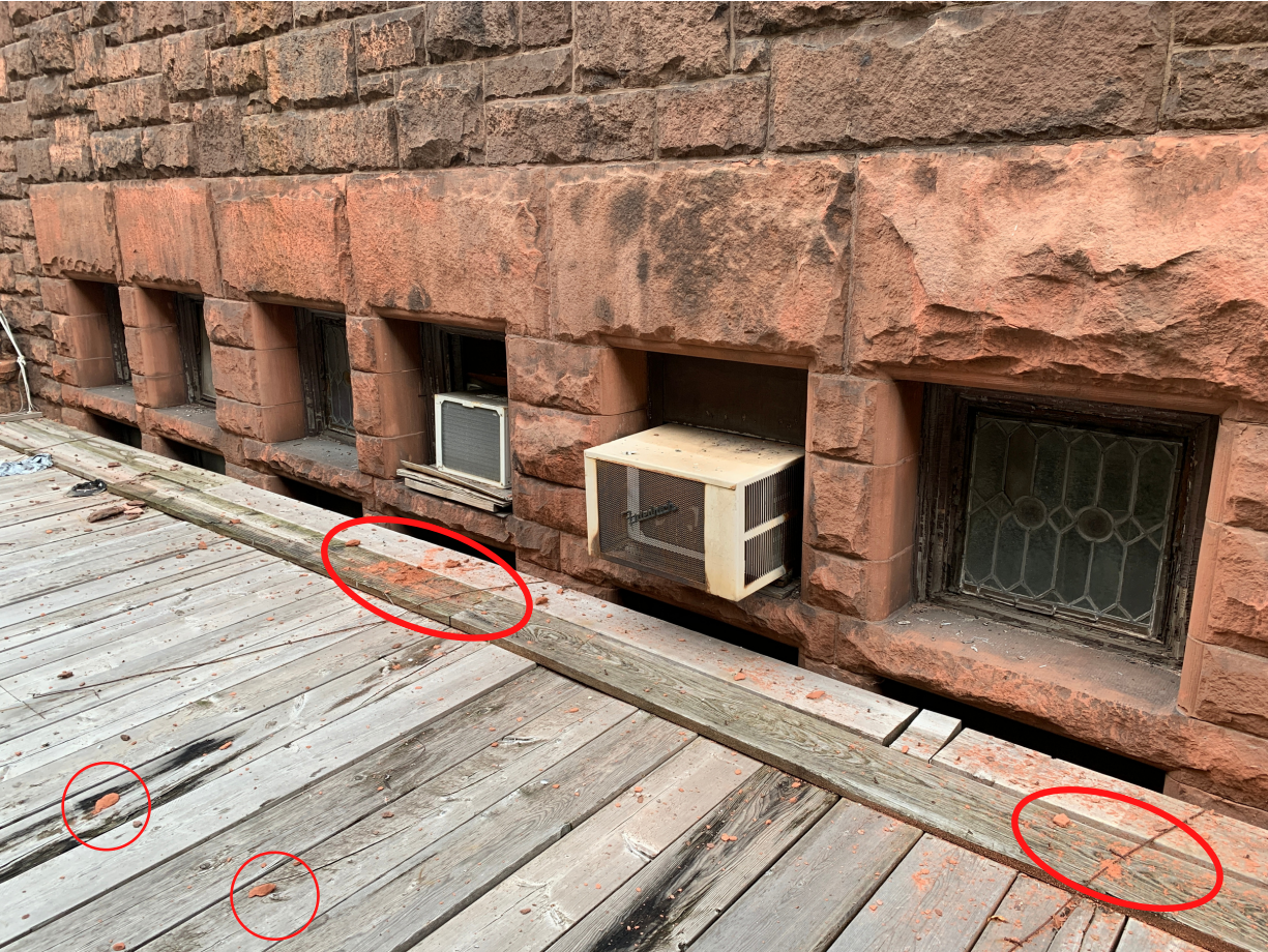
Many panels have been removed to accommodate air condition units across the building. Note the pieces of stone which have fallen on the sidewalk bridge.
