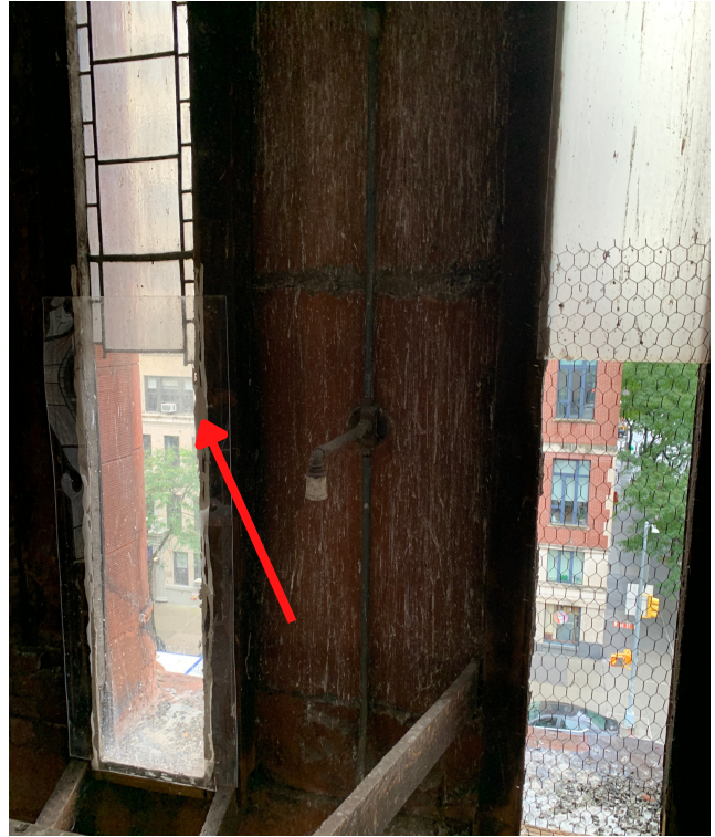
This remaining panel in danger of falling out. There is nothing supporting it from the bottom.
