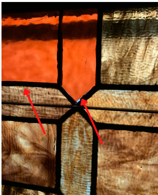
Detail of a poor repair in window S 13. The replacement glass is not a good match to the surrounding material.
