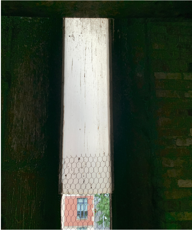
An opening with missing leaded glass that has been secured with plastic and chicken wire. This is not weather tight, and water is infiltrating the tower.
