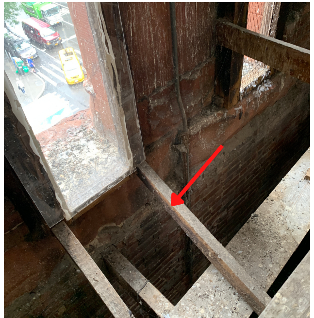
The frame appears to be shored by 2x2 lumber. The stone stool has been lost on the interior. The window frame is in danger of falling out of the setting.
