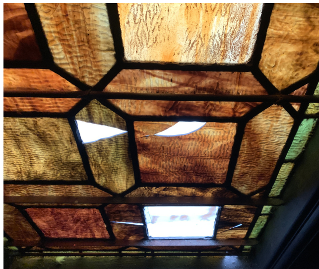
Detail illustrating several lost and unstable glass pieces in window S 13.
