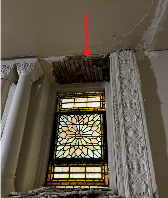
Detail of lost, cracked and damaged plaster in window N 1.
