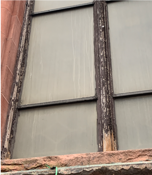
Details illustrating typical exterior wood and steel conditions. The paint has chipped away exposing bare wood and steel. The steel ventilators have rusted.
