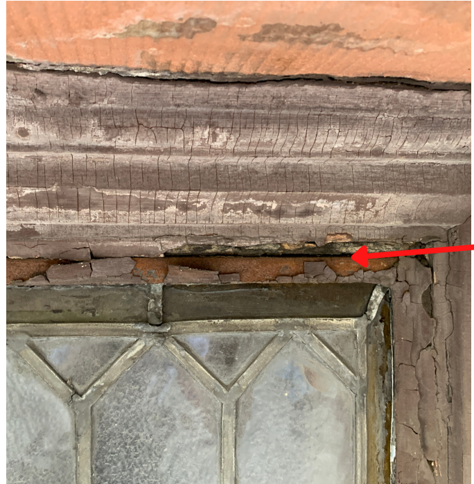
Details illustrating typical exterior wood and steel conditions. The paint has chipped away exposing bare wood and steel. The steel ventilators have rusted.
