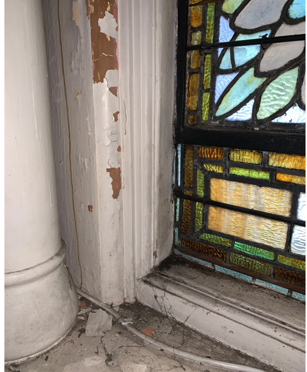
Detail of window S 9 showing chipping interior paint which is typical across the building.
