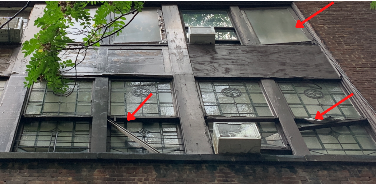
Pieces of the wood sashes and Lexan framing are in danger of falling on the northern side of the parish house. The caulk adhering the Lexan has failed and the Lexan is unstable.
