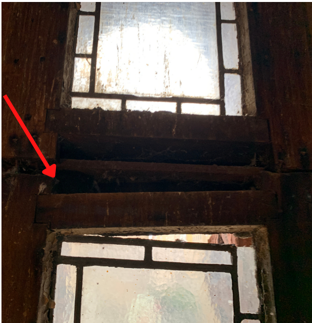
Detail of frame slippage. The top of the frame is no longer holding in the window.
