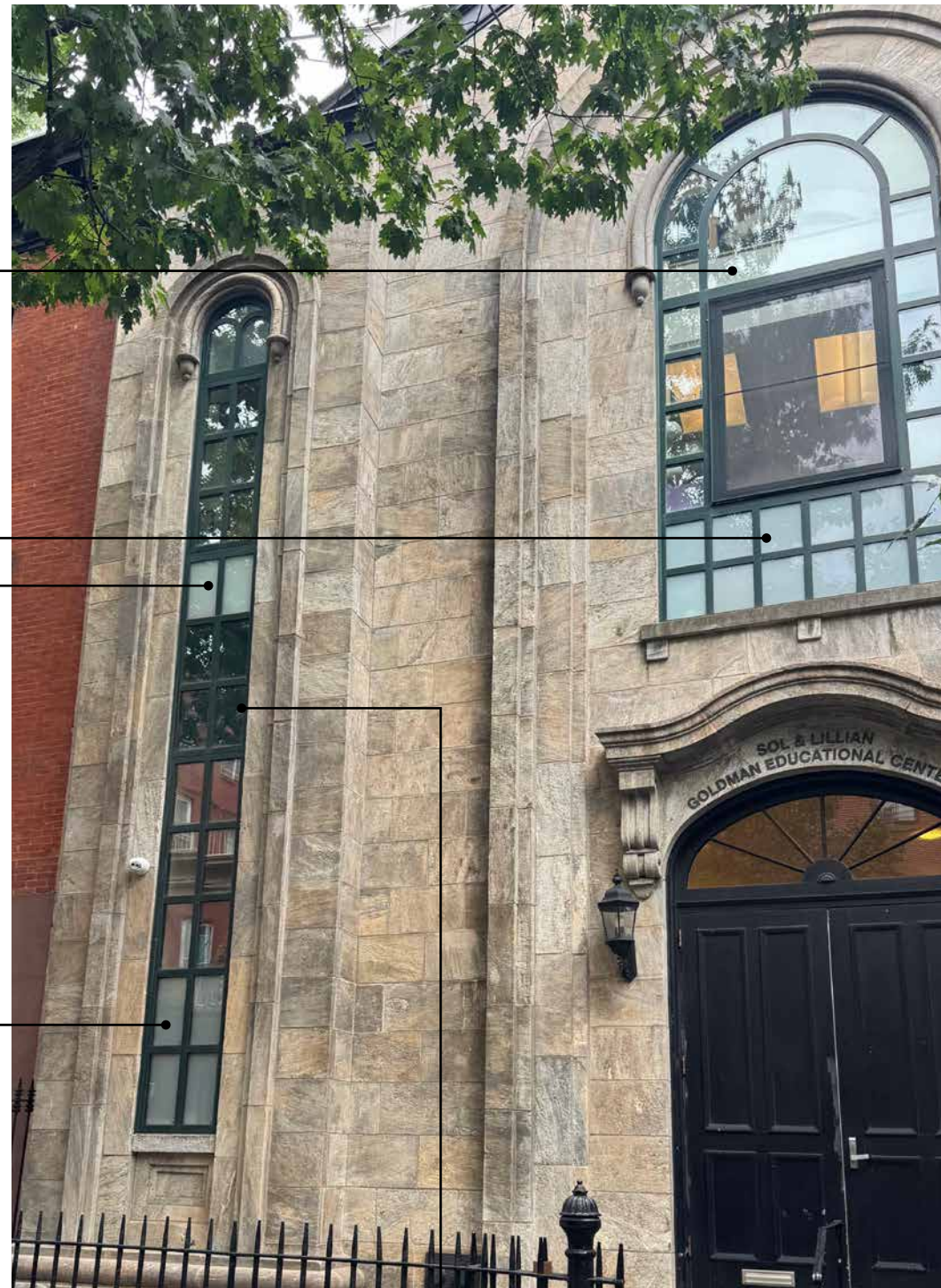
Spandrel panel at second floor
