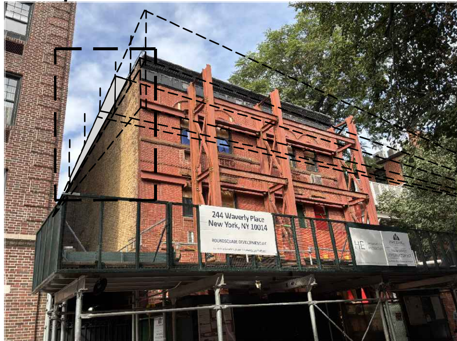
Oblique Visibility from Across Waverly Place (Towards 11th St)
