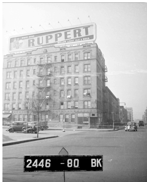
Williamsburg Bridge Approach
