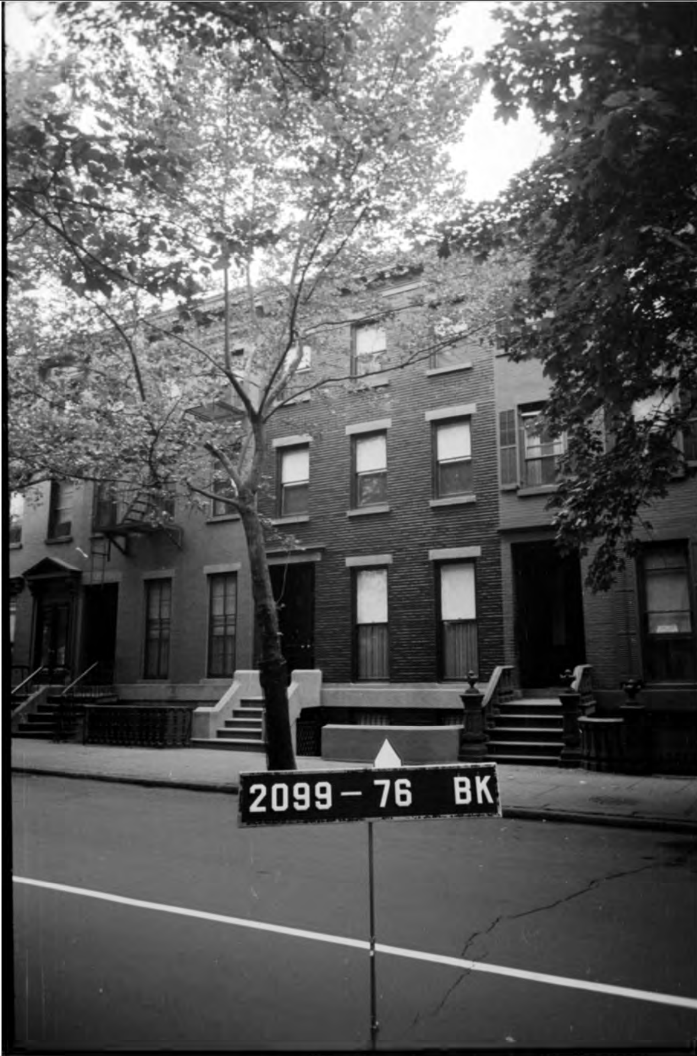
FRONT FACADE _ LPC TAX PHOTO 1940
