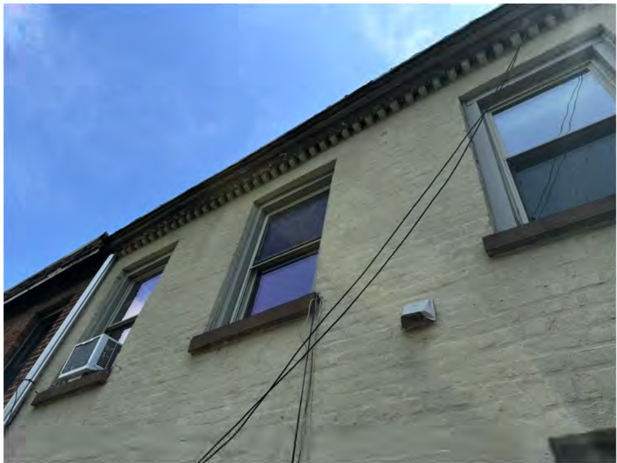
EXISTING REAR MASONRY 3RD FLOOR FACADE BRICK AND CORNICE DETAIL TO REMAIN N.T.S.
