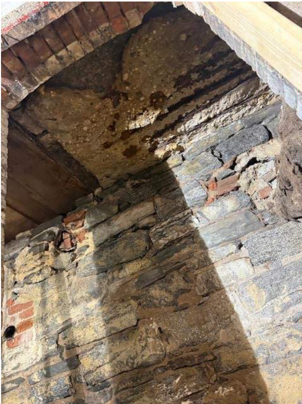
PHOTO #4 TAKEN AT THE INTERIOR OF THE VAULT FACING THE UNDERSIDE OF THE STREETSCAPE.
