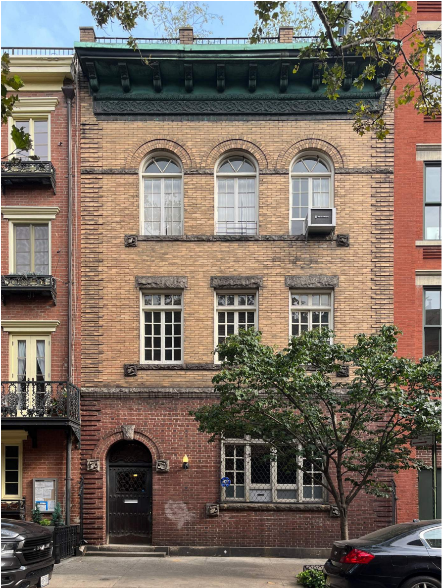
STREETSCAPE PHOTO #2 - SOUTH
