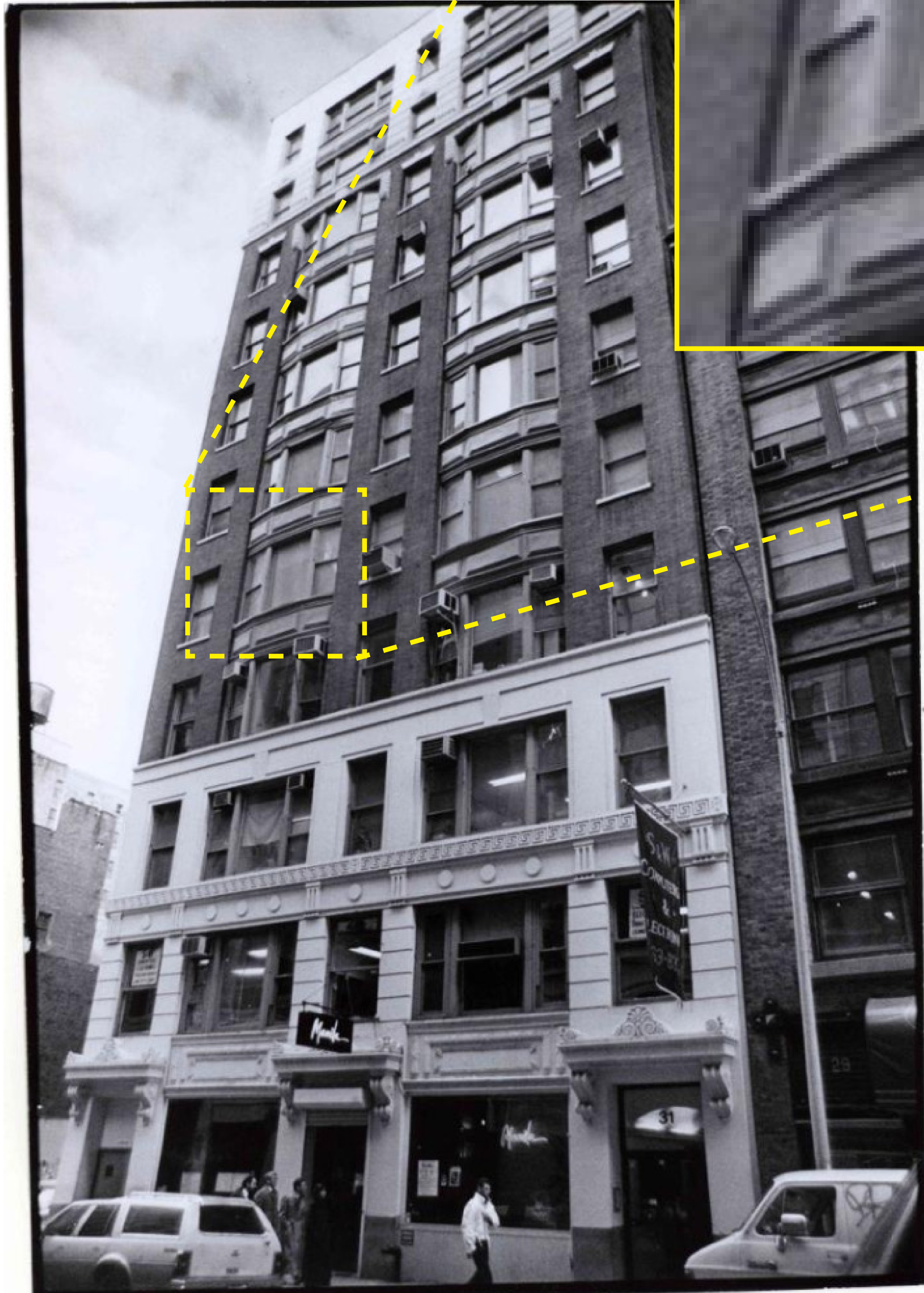
31 W 21ST STREET c.1989 @ LANDMARKS DESIGNATION “CHICAGO STYLE” DOUBLE HUNG WINDOWS ON BAY SIDES
