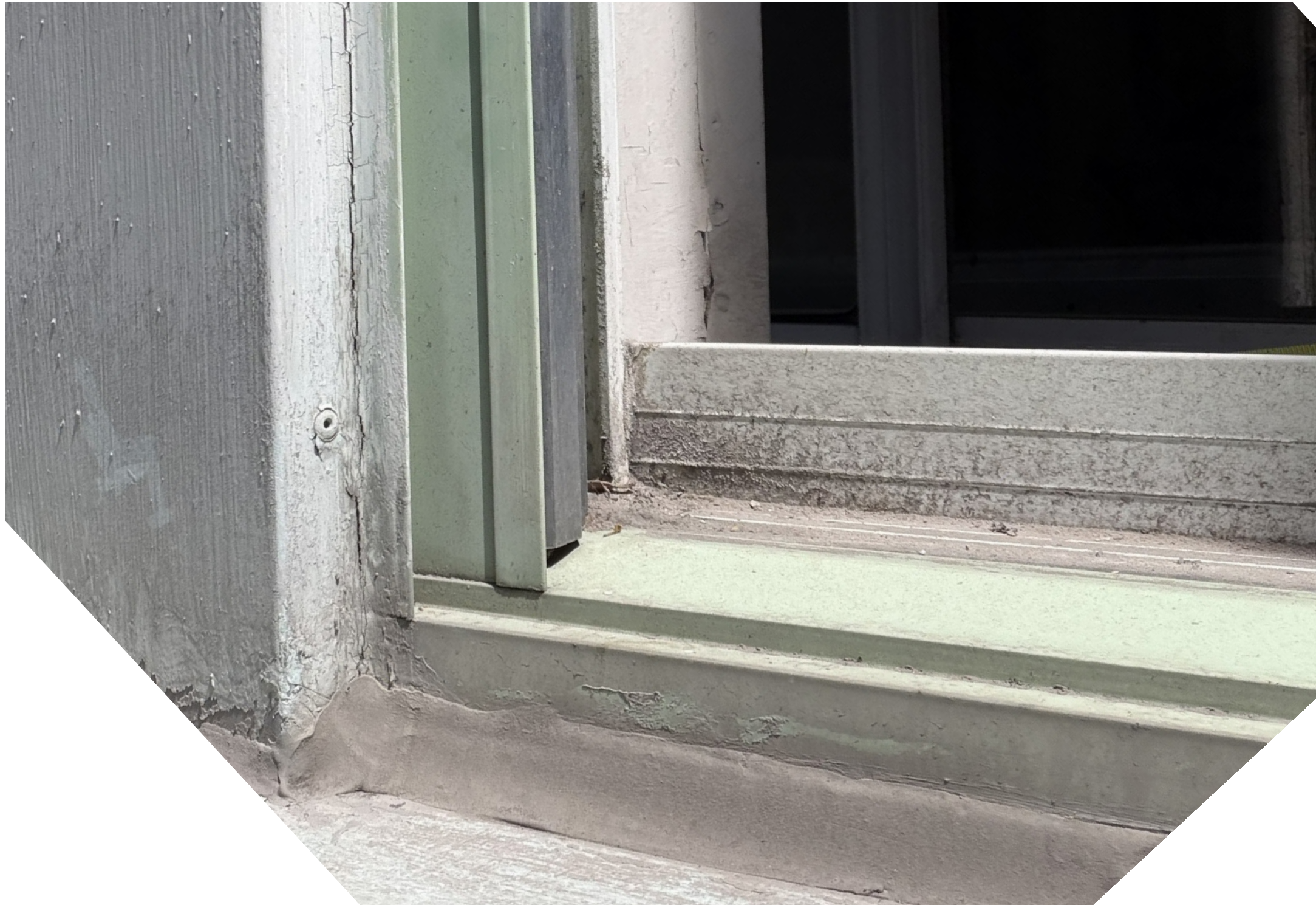
METAL MULLION CAP RELATIONSHIP TO EXISTING WINDOW | SILL DETAIL | EXISTING WINDOW PROFILES
