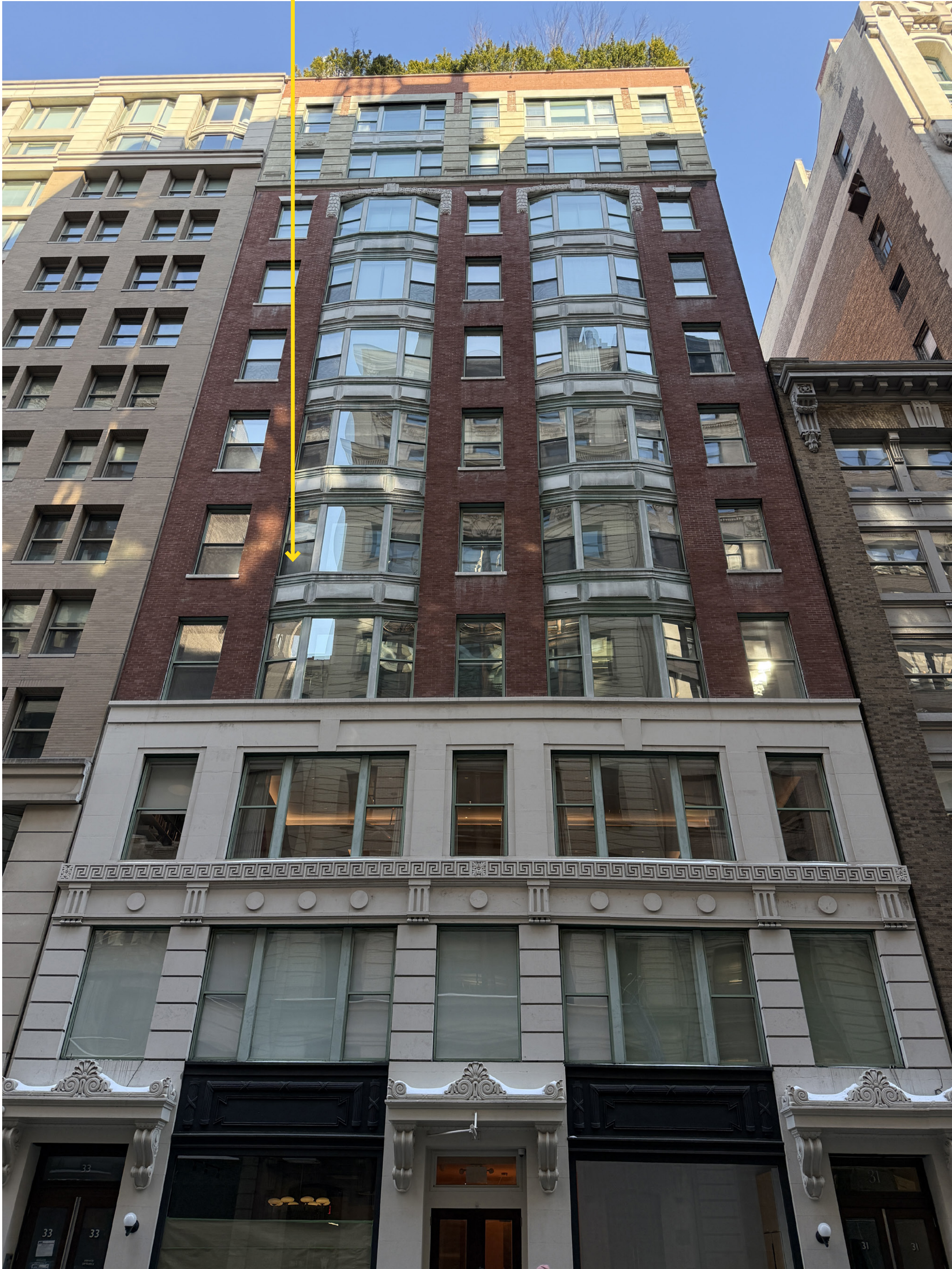
31 W 21ST STREET c. 2026(EXISTING)
