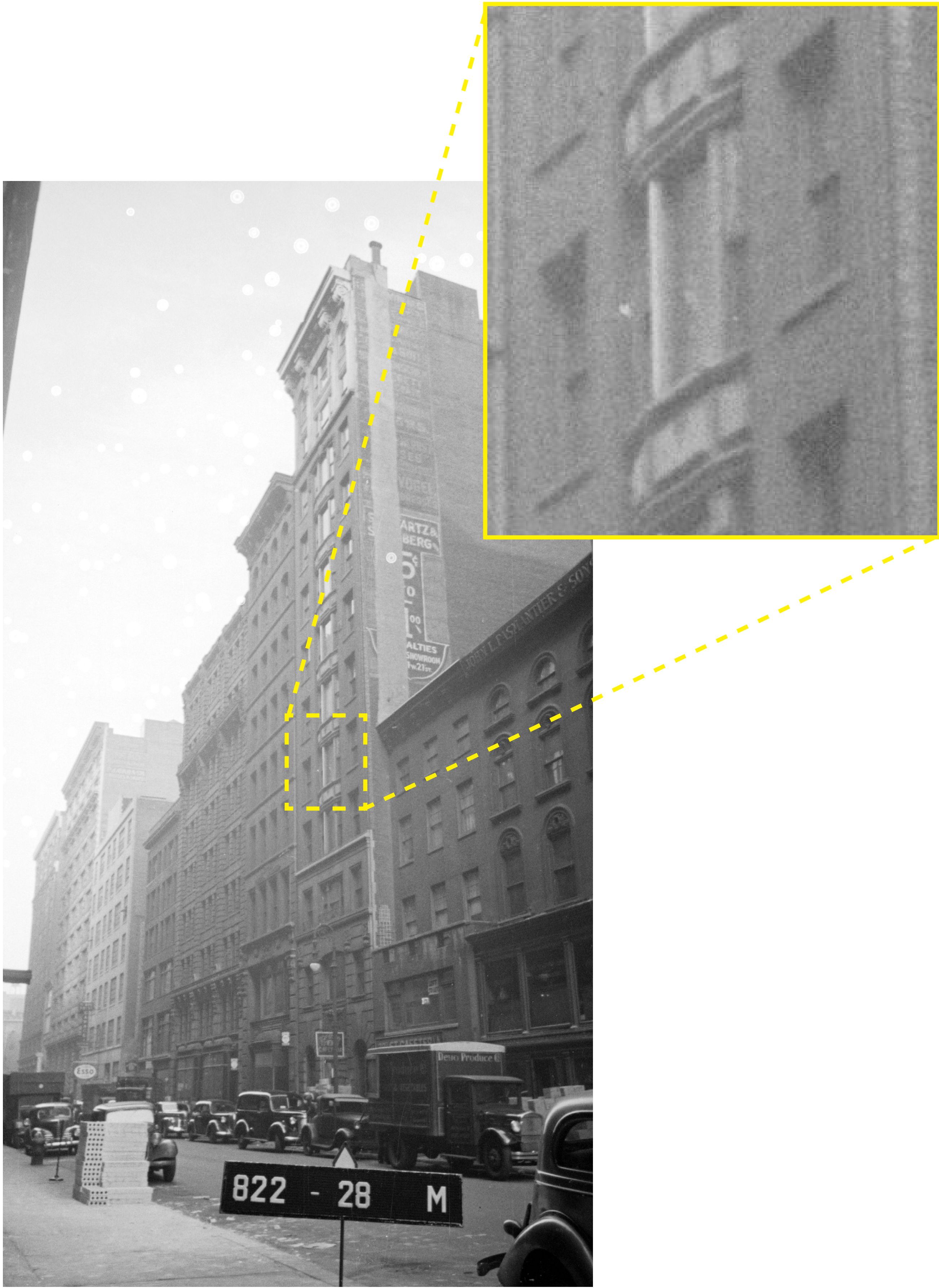
9 W 20TH STREET C. 1940 CHICAGO STYLE BAY WINDOWS W/ METAL SPANDREL
