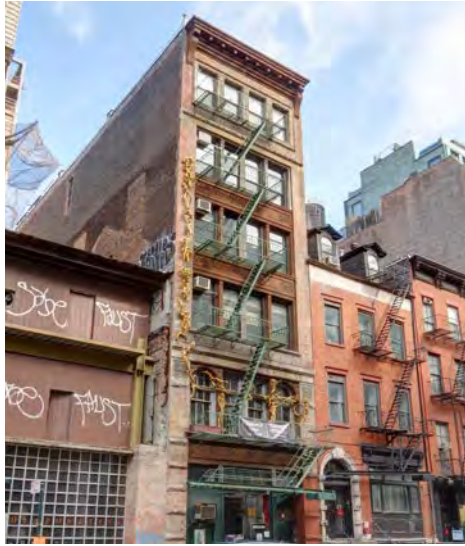
24 Bond St. Robert Maplethorpe's Residence
