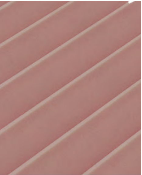
Corrugated Aluminum Bulkhead Siding Painted to Match Facade
