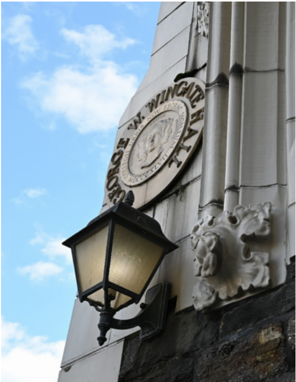
Decorative terra cotta, ironwork, seal
