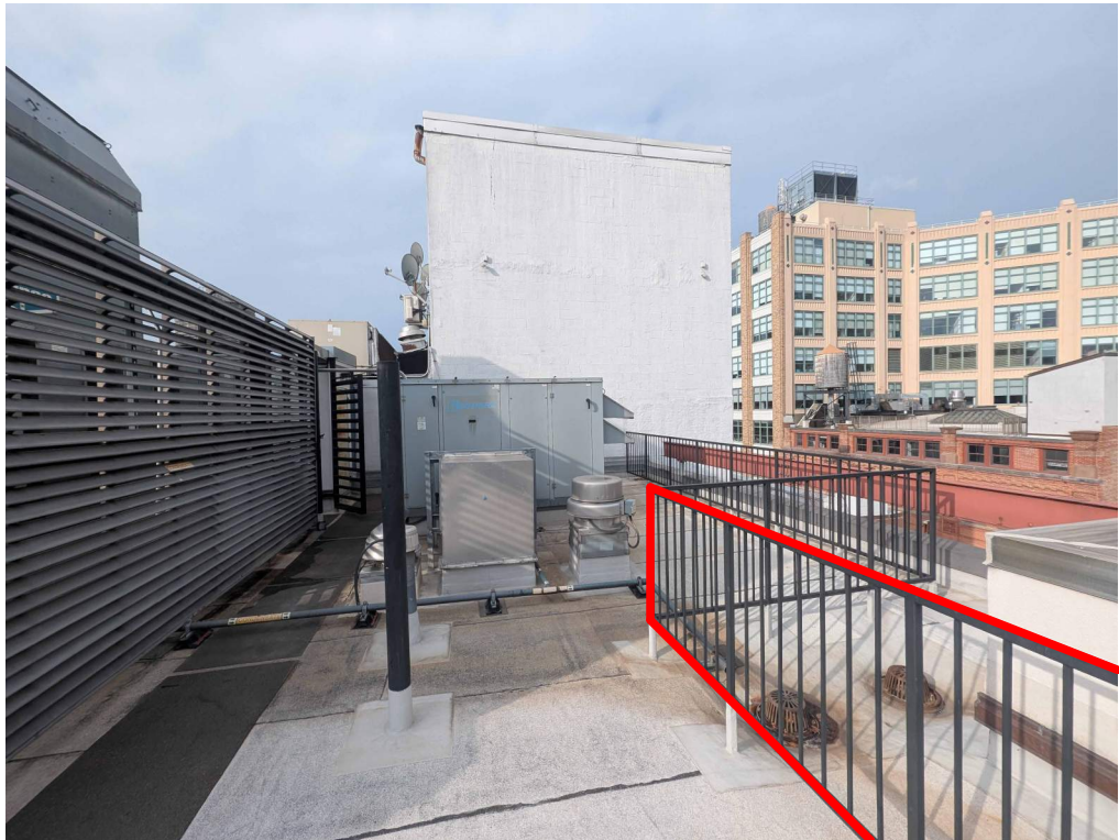
20 EXISTING RAILING ON ROOF- RED HIGHLIGHTED SECTION TO RELOCATE
