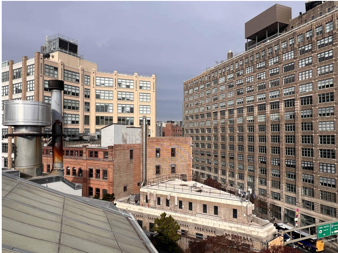
11 VIEW OF SURROUNDING ROOFTOPS WITHIN HISTORIC DISTRICT
