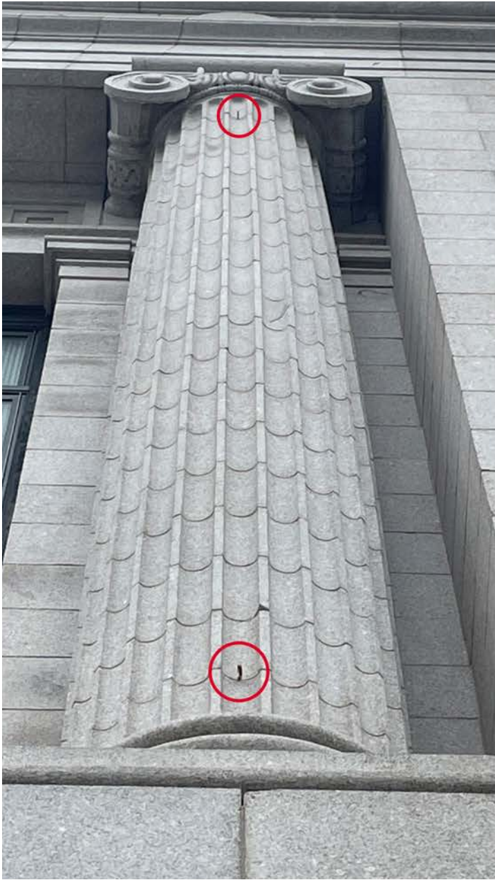
TYPICAL EXISTING CLOSED-EYE ROUTING EYEBOLT HARDWARE AT COLUMN OF EAST FACADE TO REMAIN AT ALL LOCATIONS
