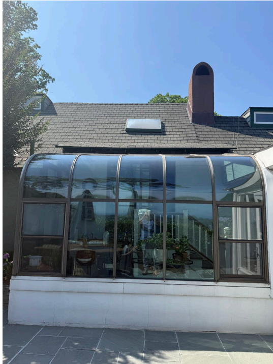
Skylight to be removed.
