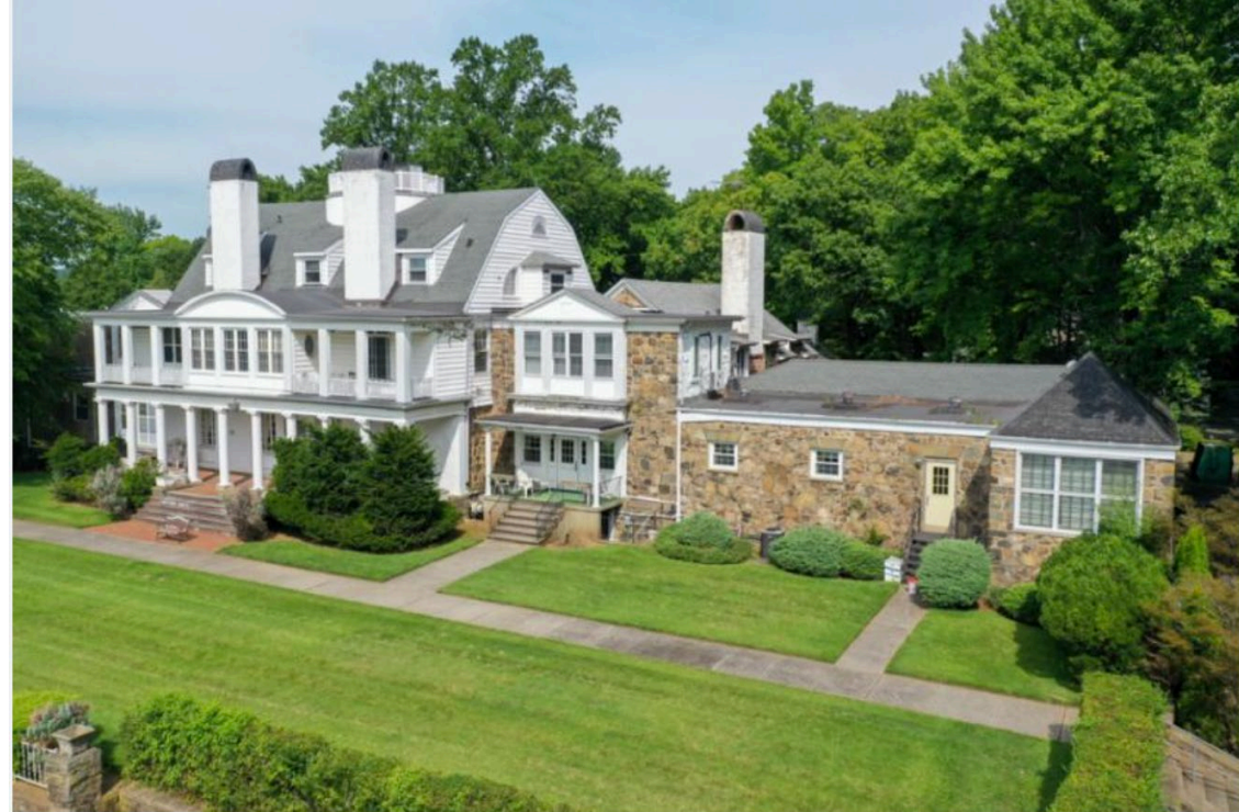
Flaggs main house shows 3 different types of construction on 3 porches, brick, cement, and iron.
