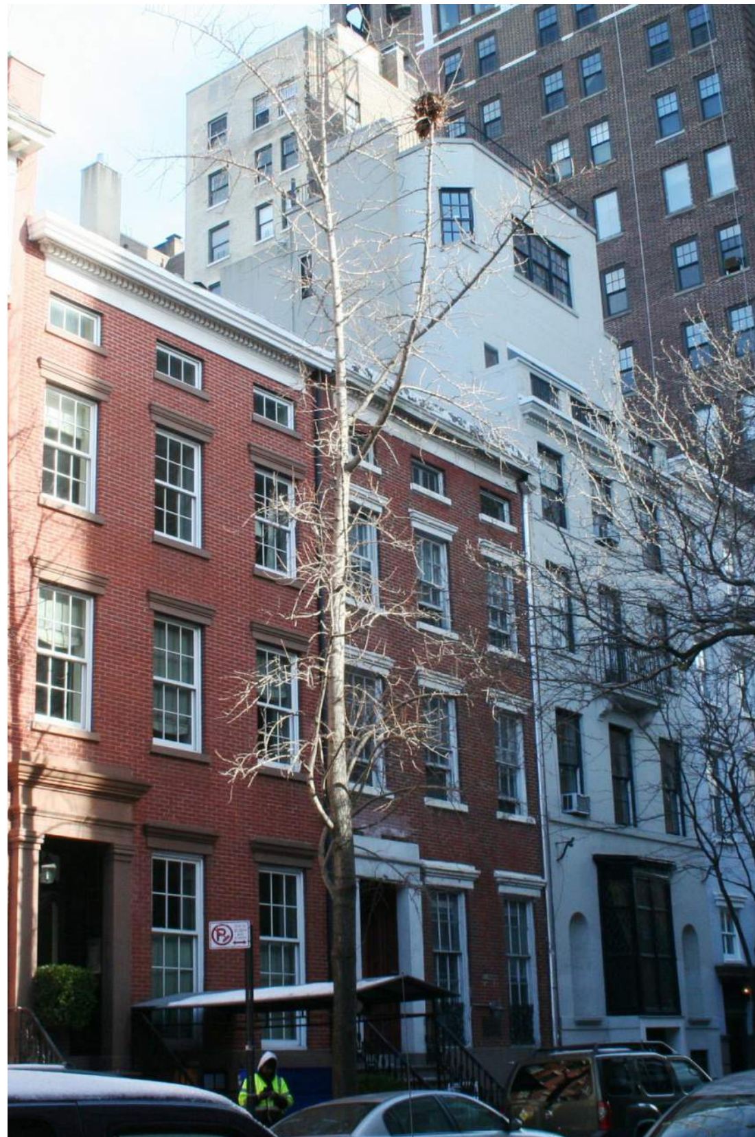
PHOTOGRAPH - FRONT FACADE (SOUTH) - 2015
