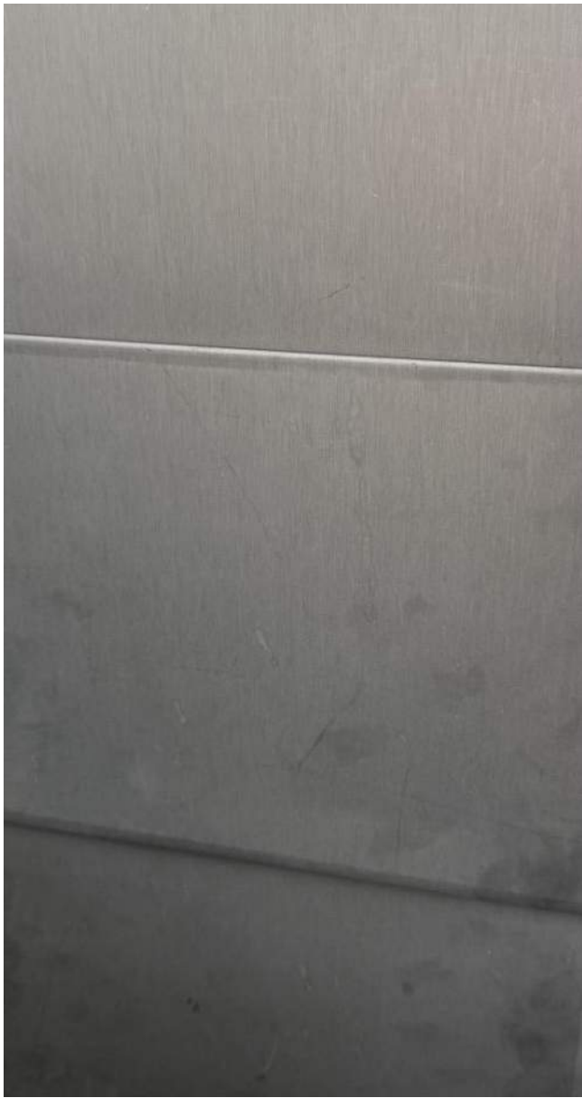
PENTHOUSE CLADDING - ZINC SHINGLES
