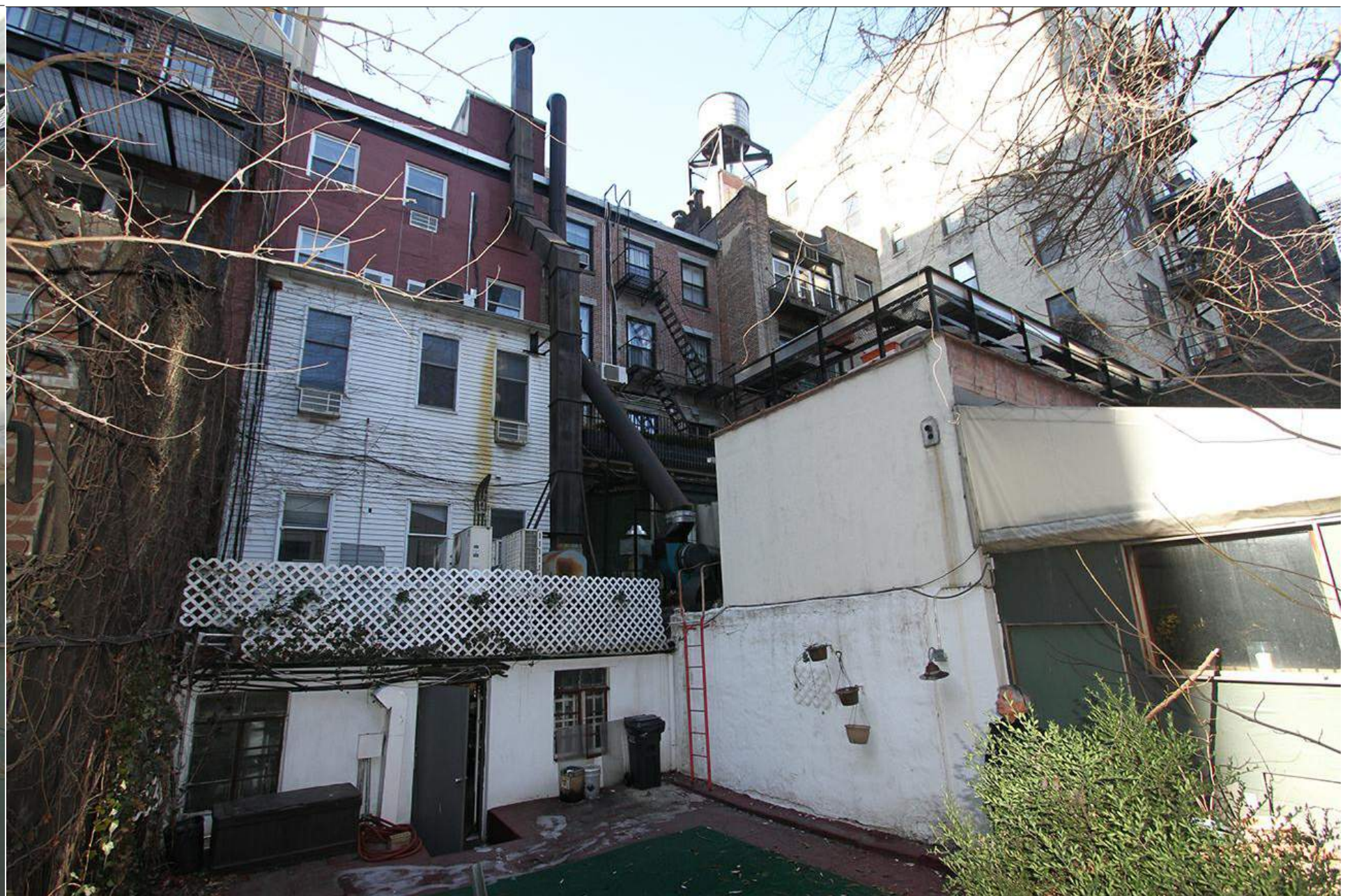
PHOTOGRAPH - NEIGHBOR'S FACADE (NORTH)
