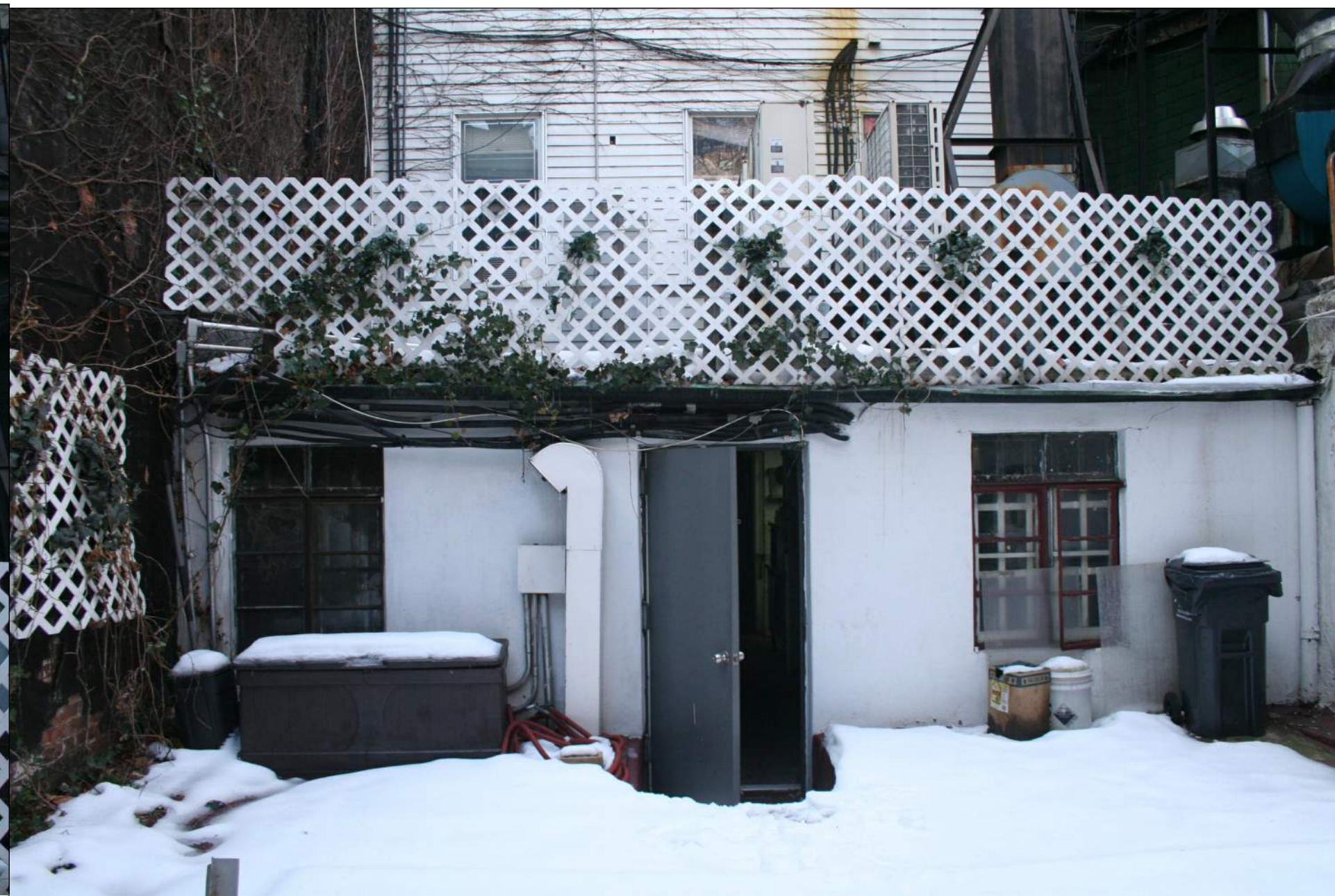
PHOTOGRAPH - REAR FACADE
