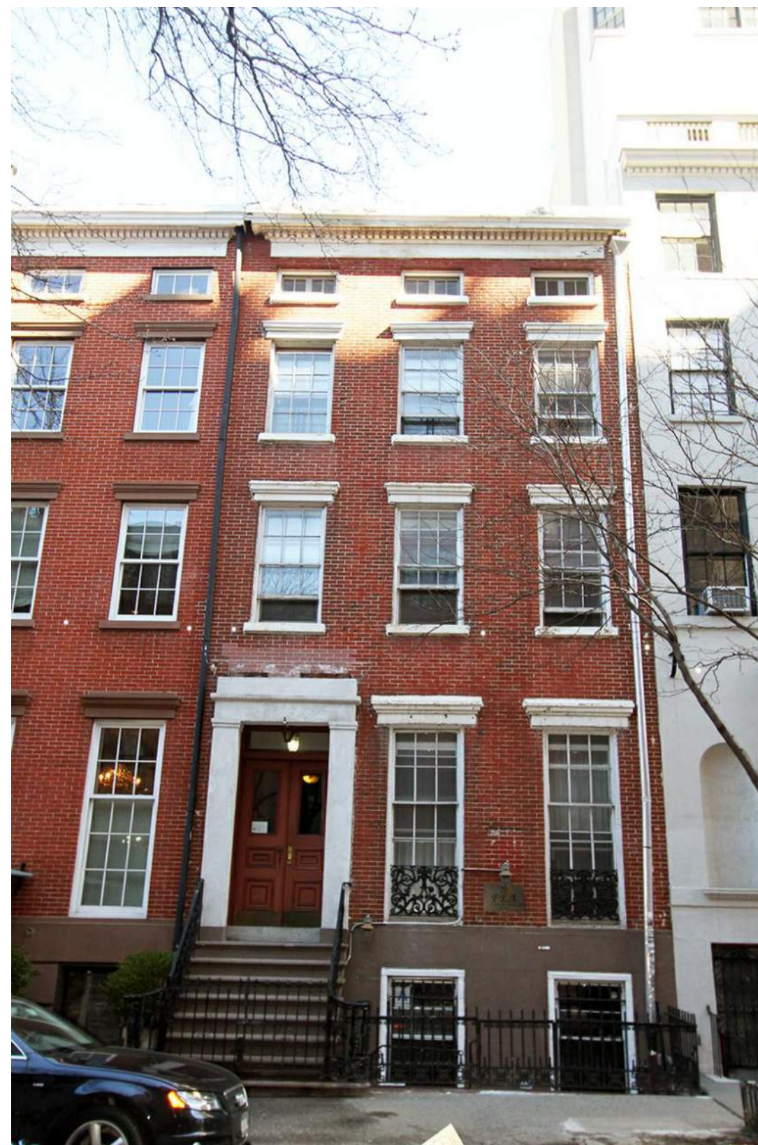
PHOTOGRAPH - FRONT FACADE (SOUTH) - 2015
