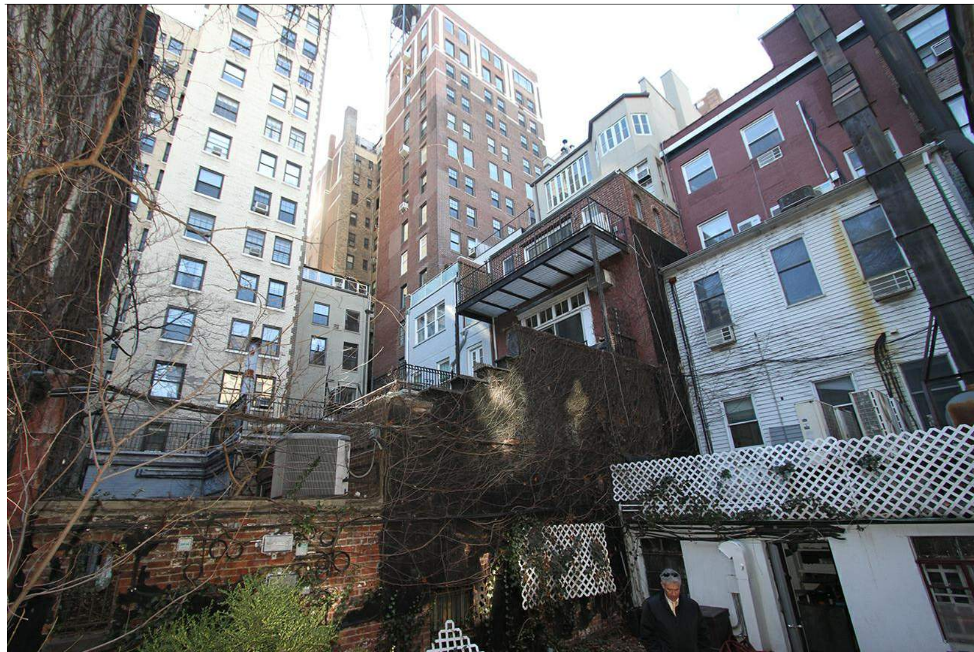
PHOTOGRAPH - NEIGHBOR'S FACADE (NORTH)
