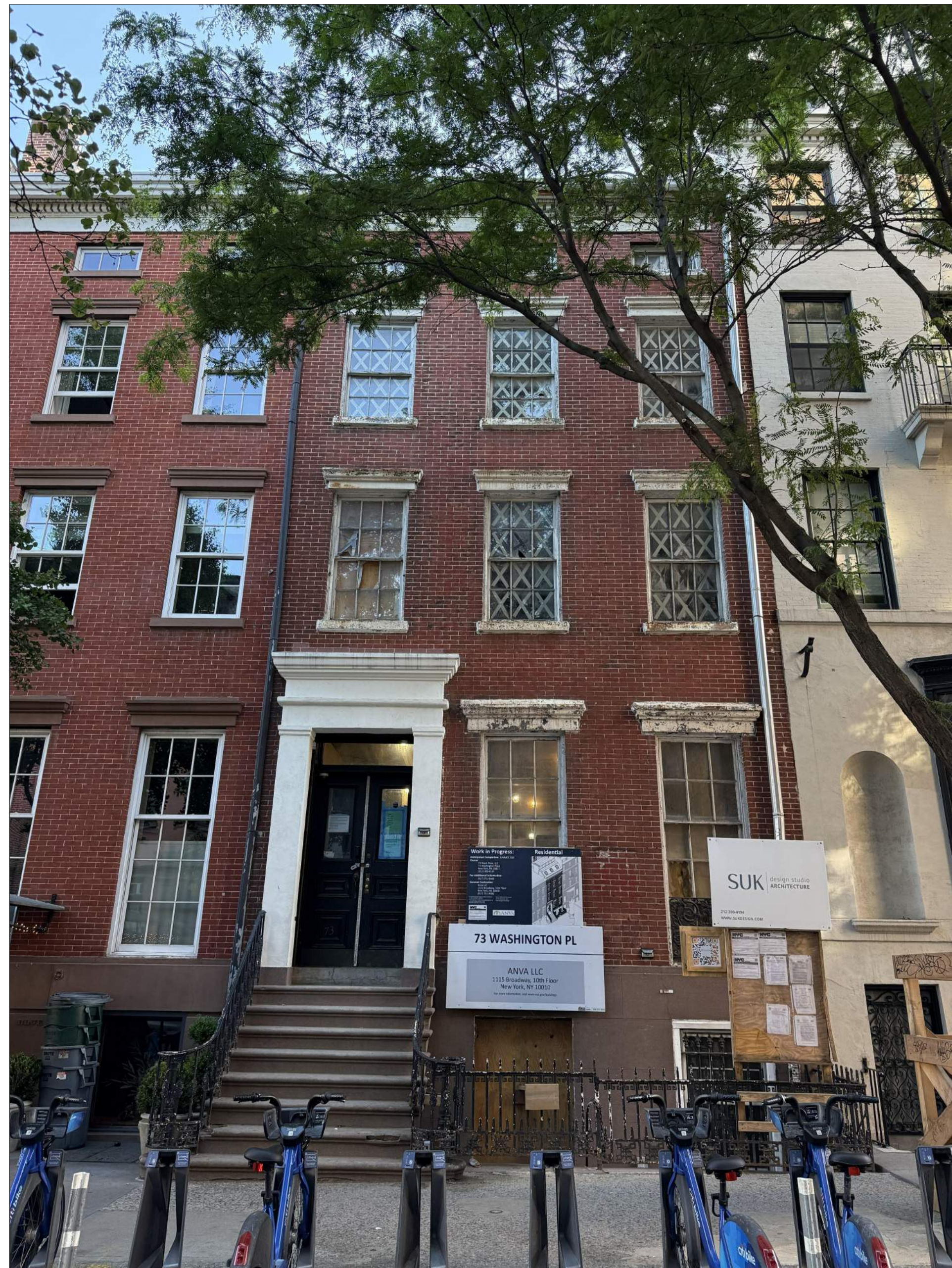
PHOTO - FRONT FACADE
