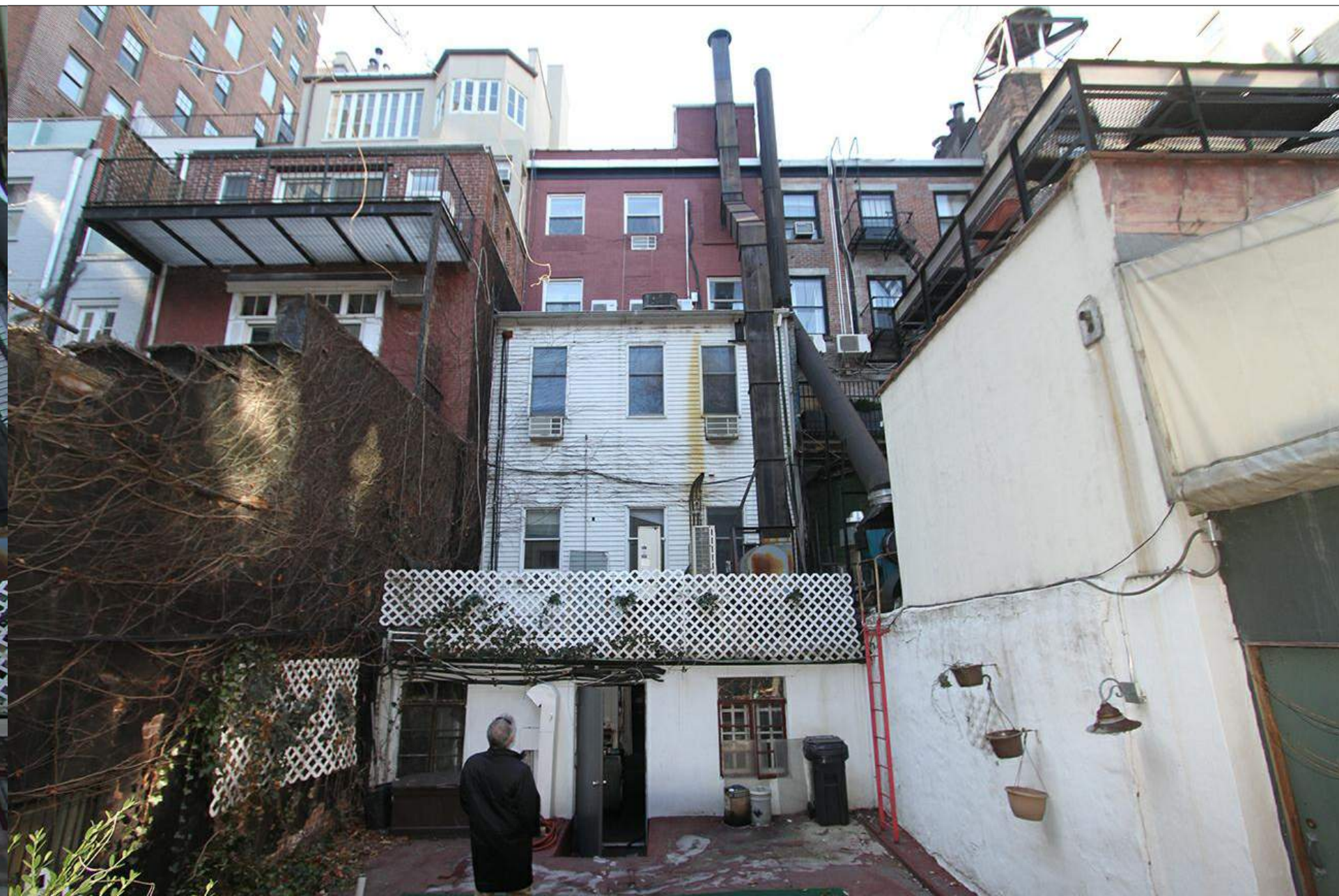
PHOTOGRAPH - REAR FACADE (NORTH)
