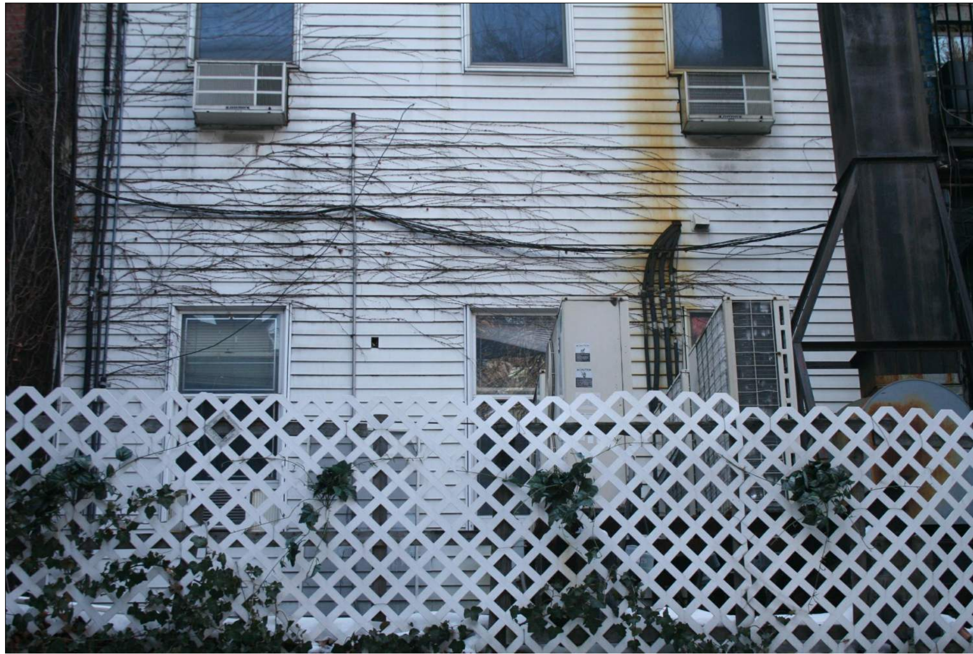
PHOTOGRAPH - REAR FACADE
