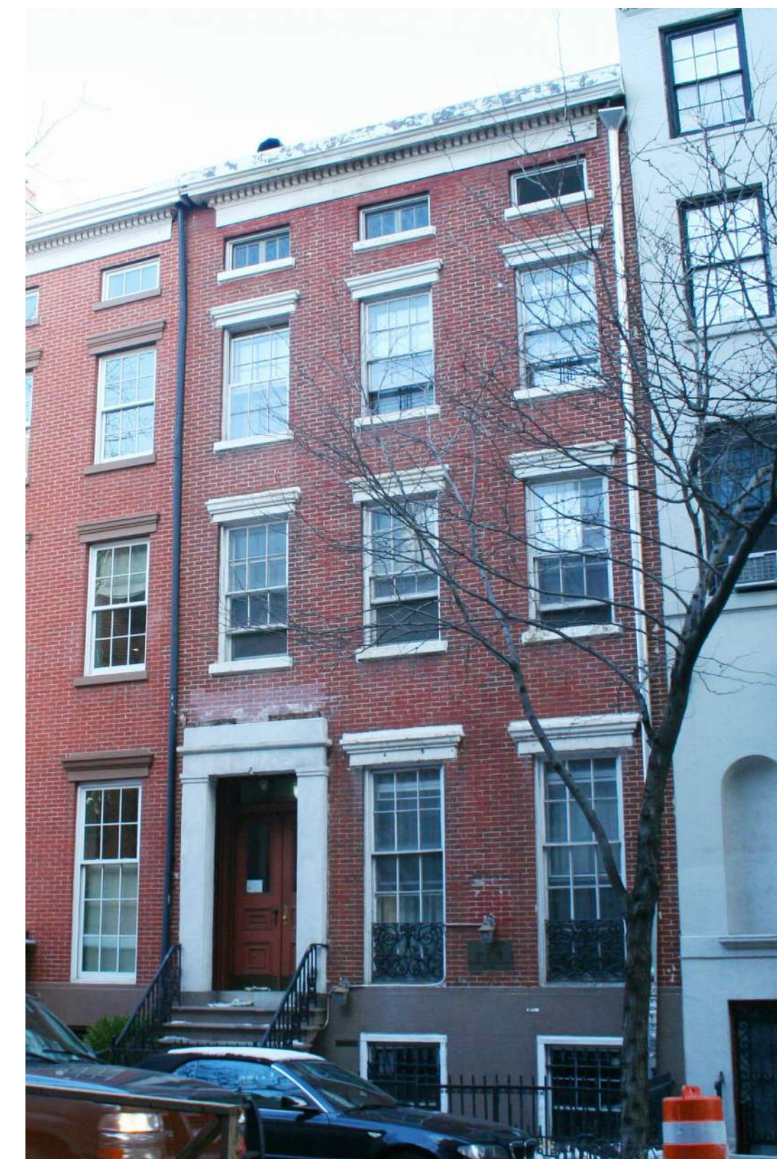
PHOTOGRAPH - FRONT FACADE (SOUTH) - 2015
