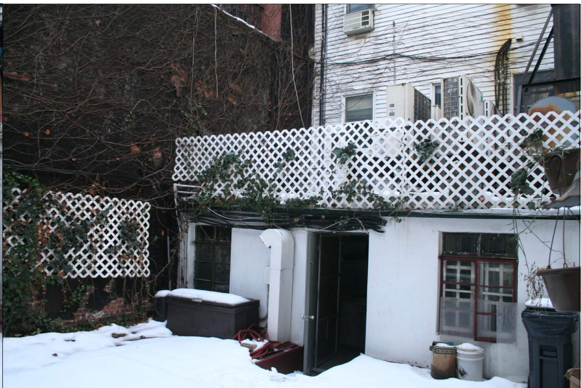
PHOTOGRAPH - REAR FACADE
