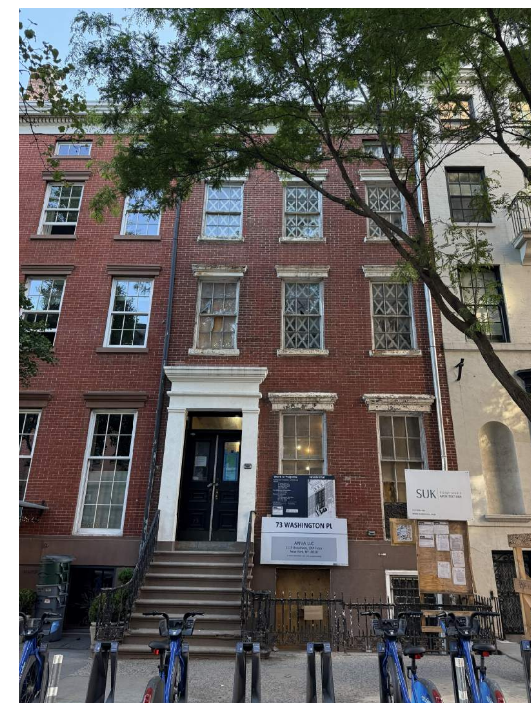
PHOTOGRAPH - FRONT FACADE (SOUTH) - JUNE 2026
