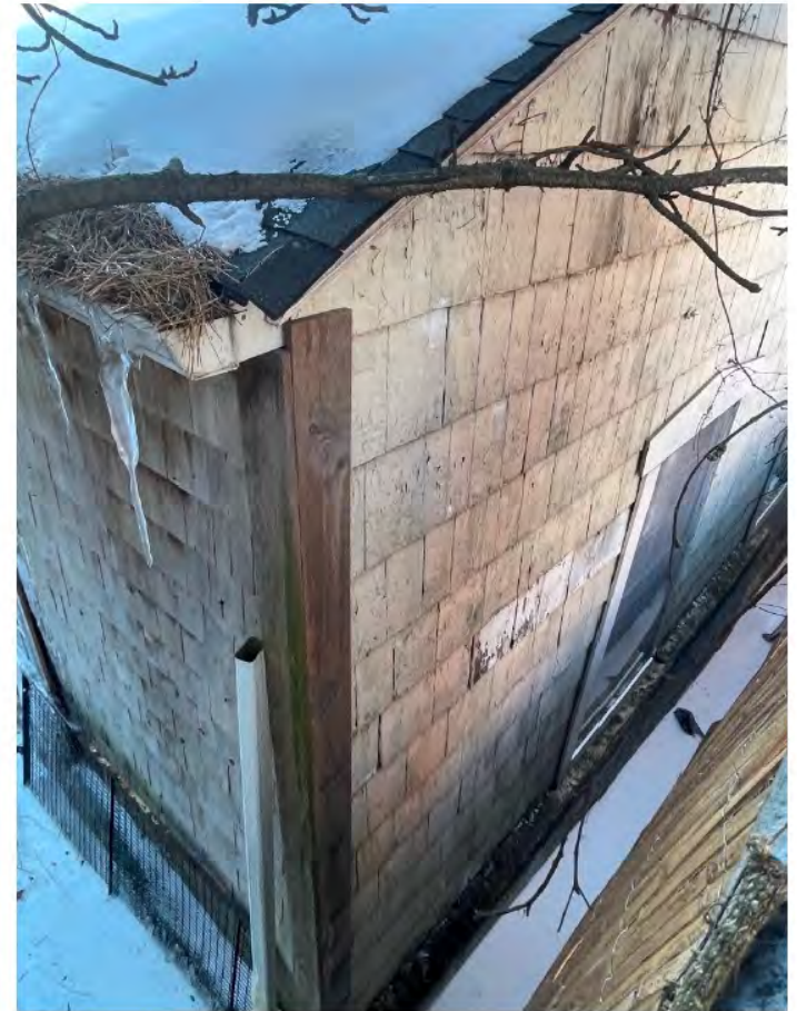
Rear facade cedar shingle installation, current condition.
