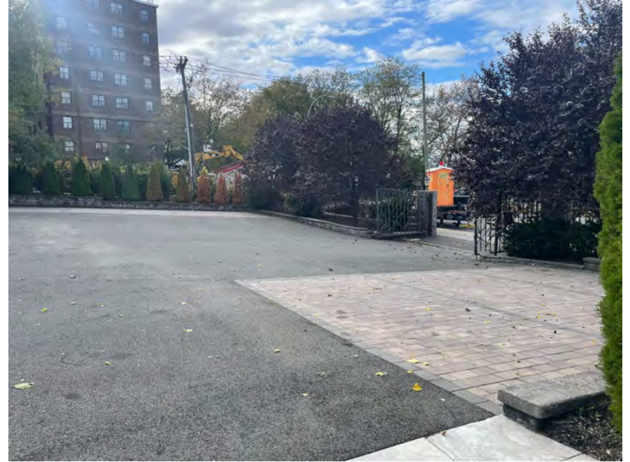
Parking area and perimeter landscaping, current condition.
