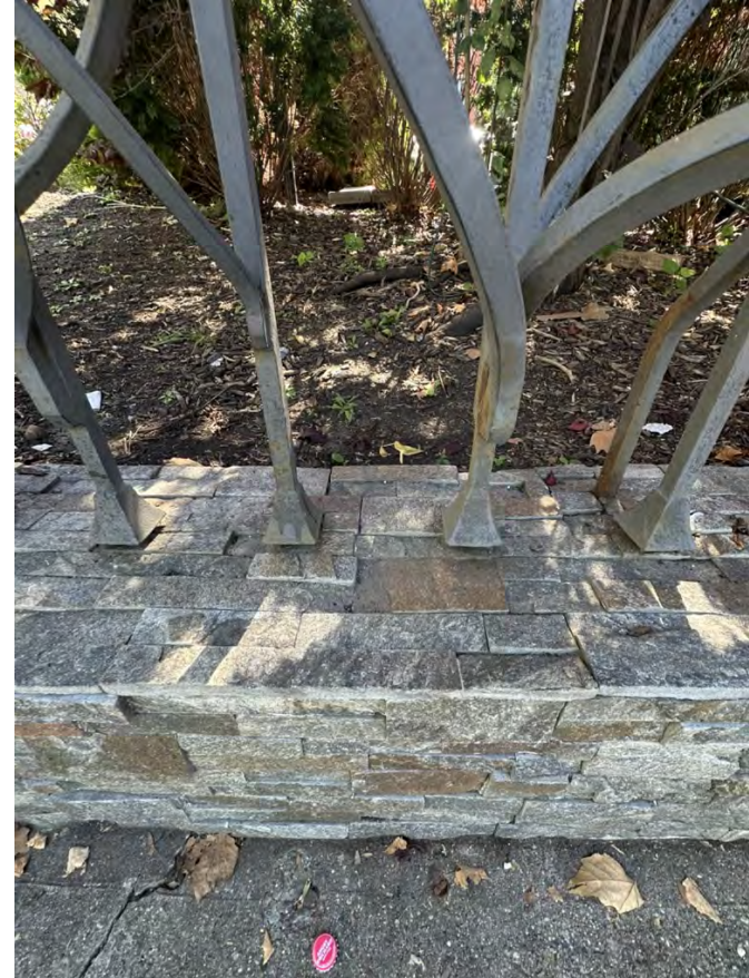
Close-up of tile-clad wall and decorative ironwork, current condition.
