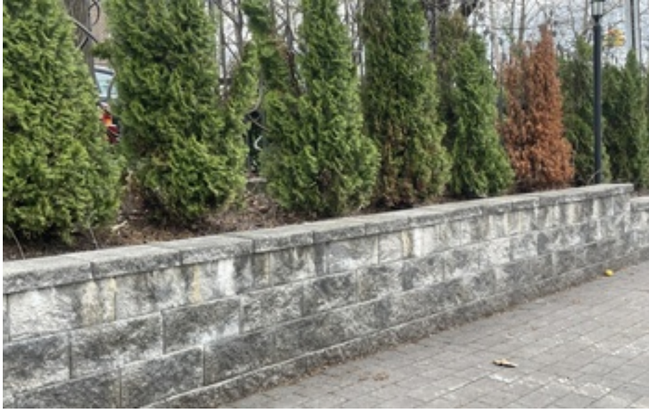
Concrete-block wall with capstone along Westervelt Avenue.
