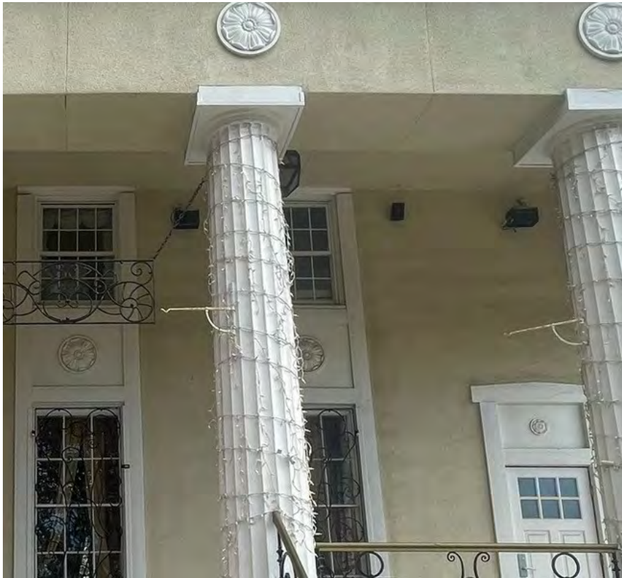
Exterior building-mounted fixture detail, primary facade.
