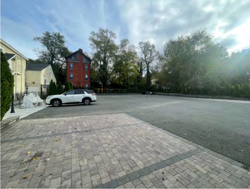
Parking area, current condition.
