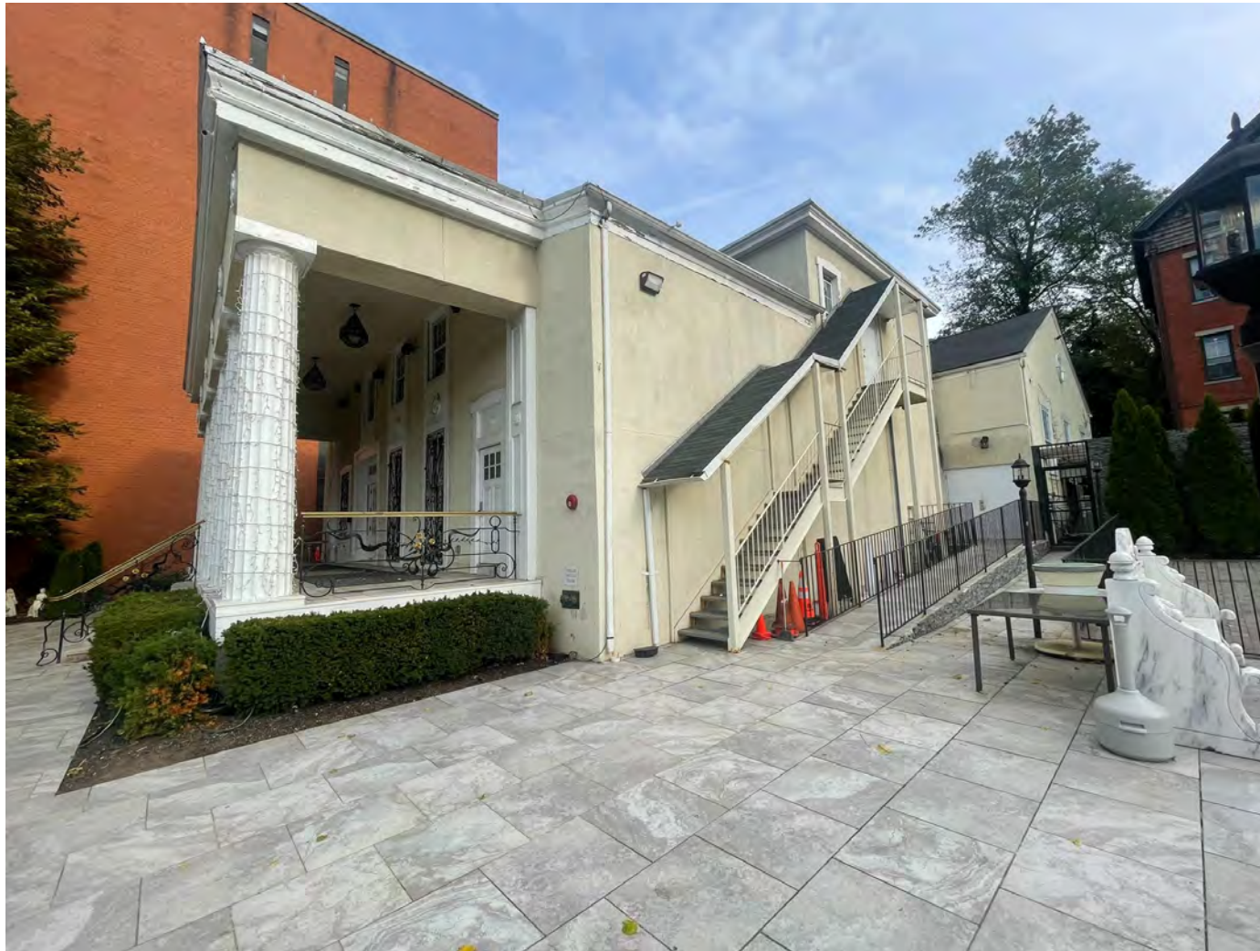
Side elevation showing exterior building-mounted lighting, current condition.
