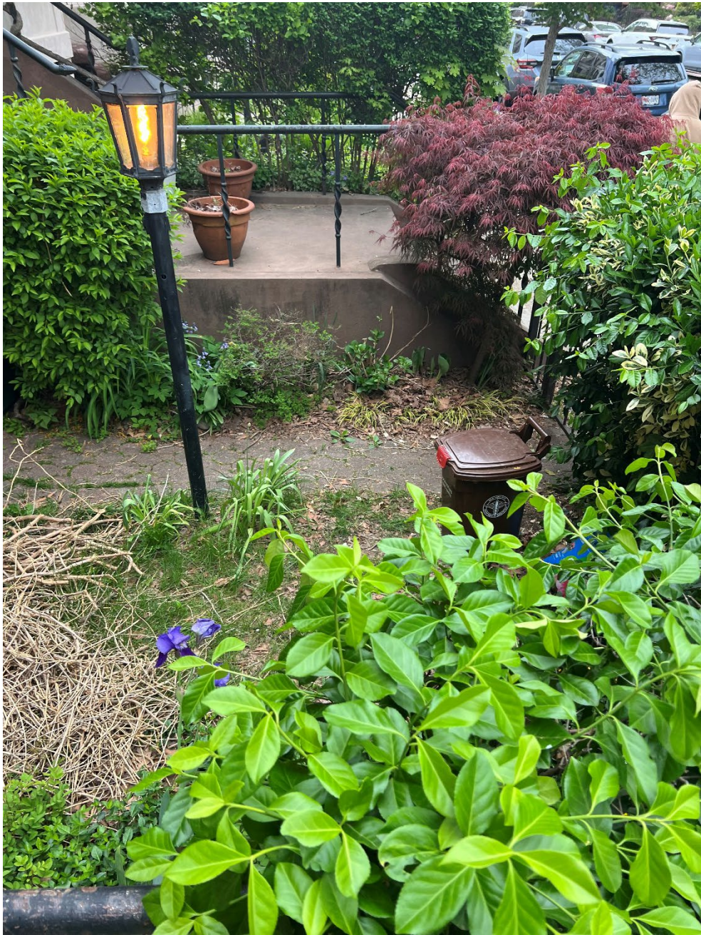
Cheek wall with stucco finish and railing
