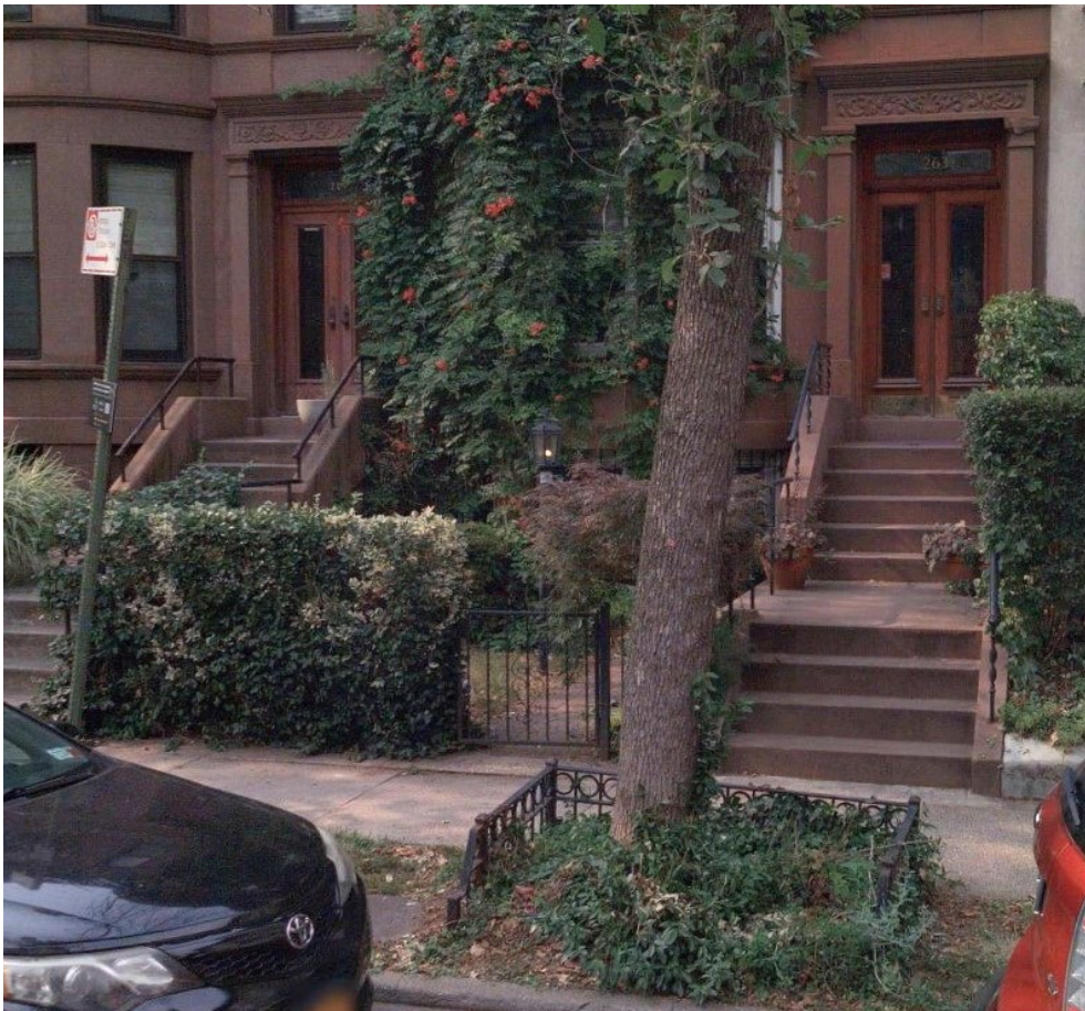
263 Sterling Street – lowered areaway
