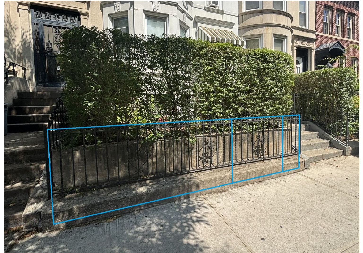
New fence in matching design and height with 42" wide gate
