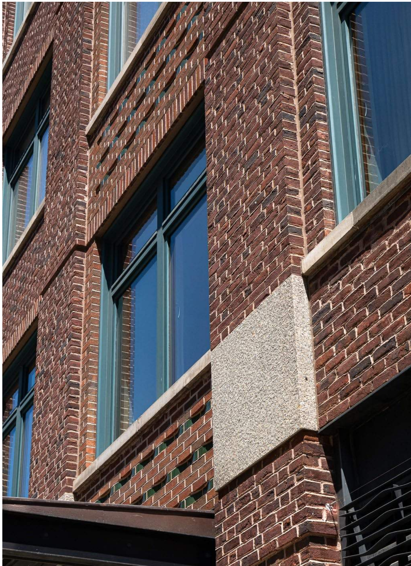
138 READE STREET (BKSK ARCHITECTS)
