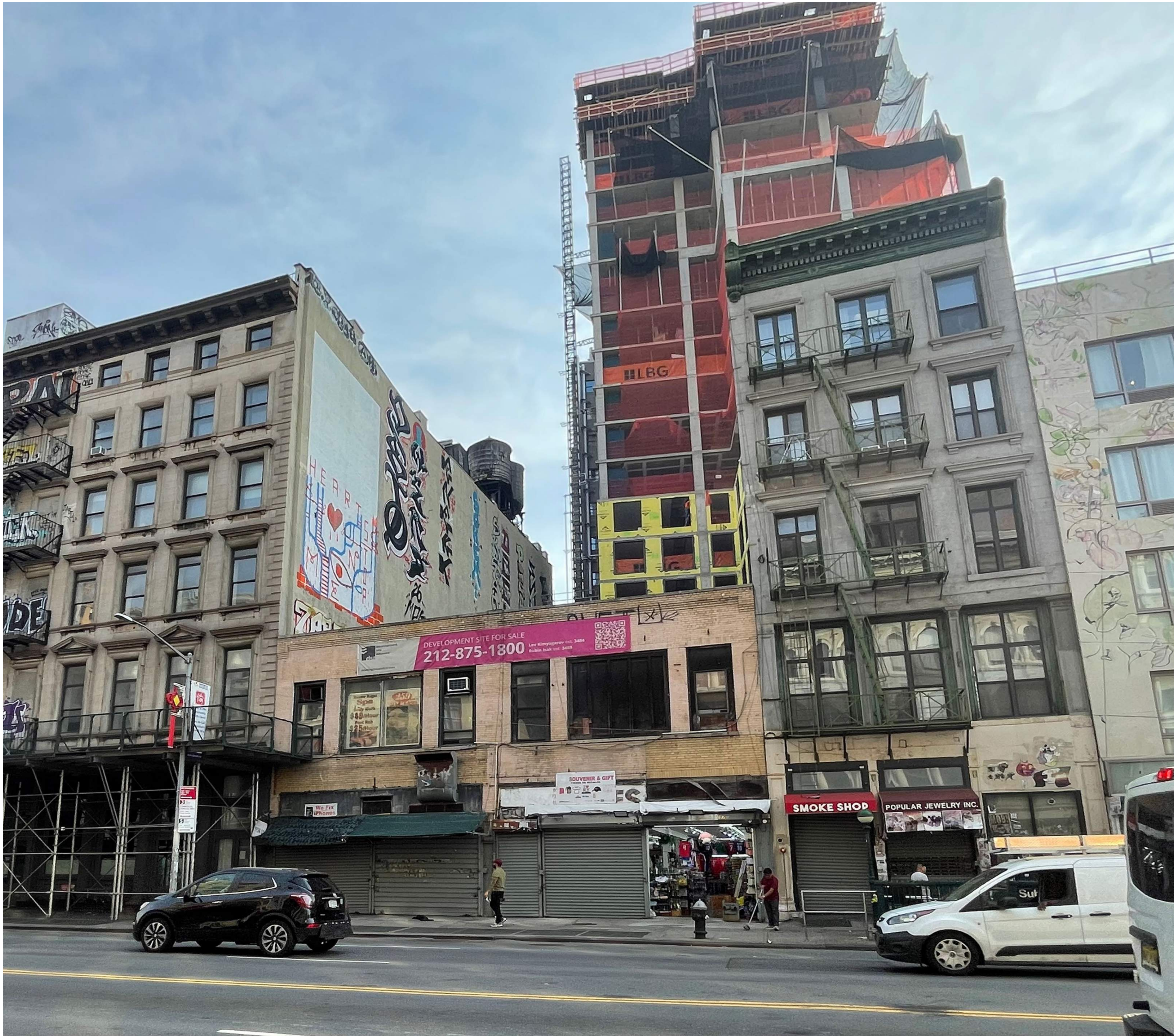
EXISTING SITE CONDITIONS
